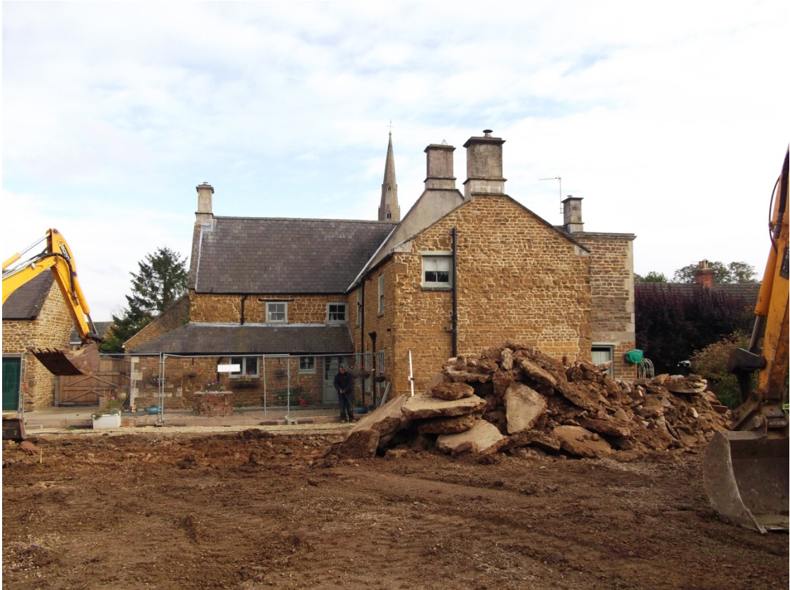
Somerby House Farm and the investigation area, looking east Fig 3
