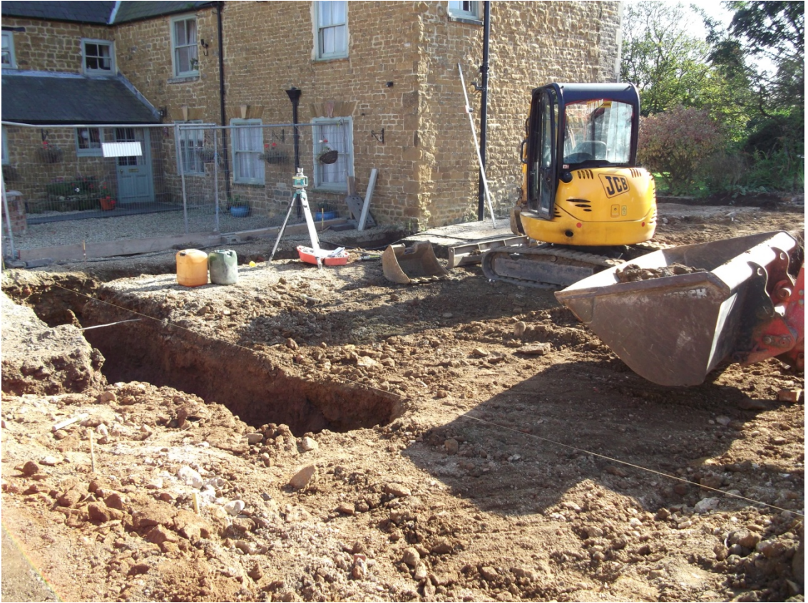
General view of the groundworks in progress, looking south-east Fig 4
