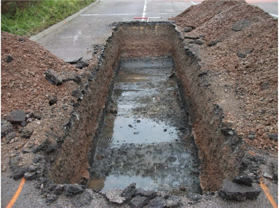
Trench 1, looking east Fig 3
