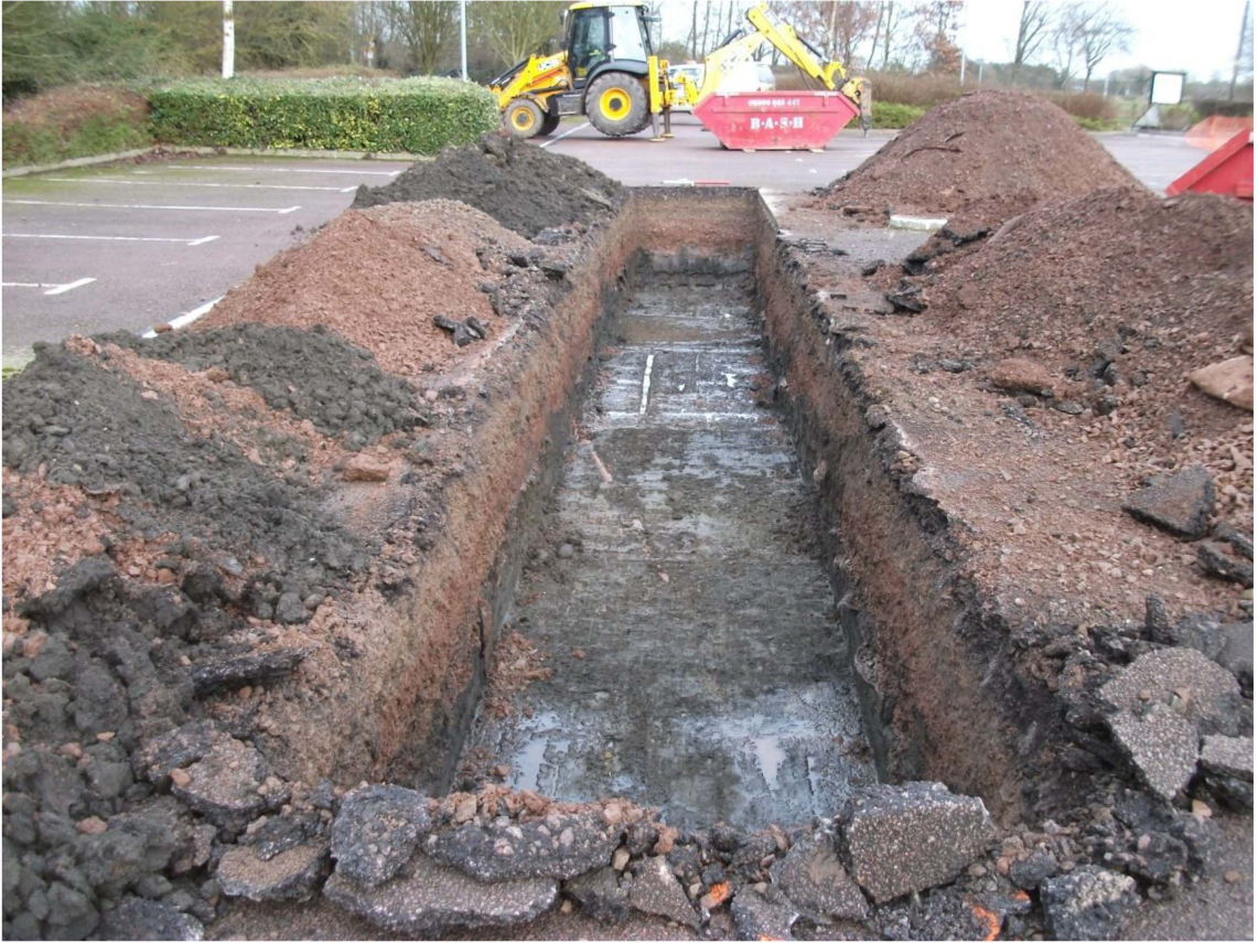
Trench 2, looking north Fig 6
