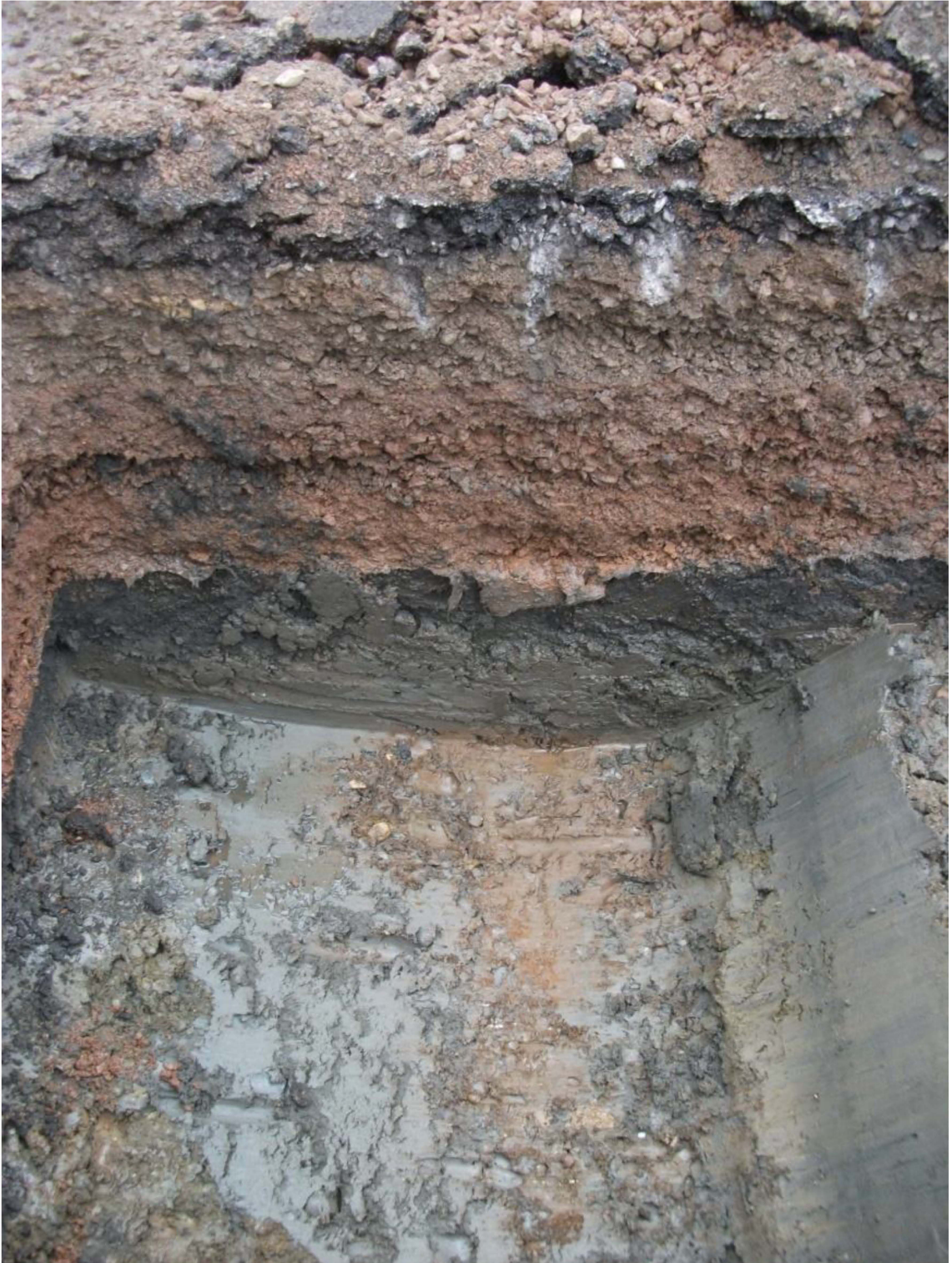
Western end of Trench 1, deepened to locate the top of the solid geology, encountered at 1.50m below the modern ground surface Fig 5
