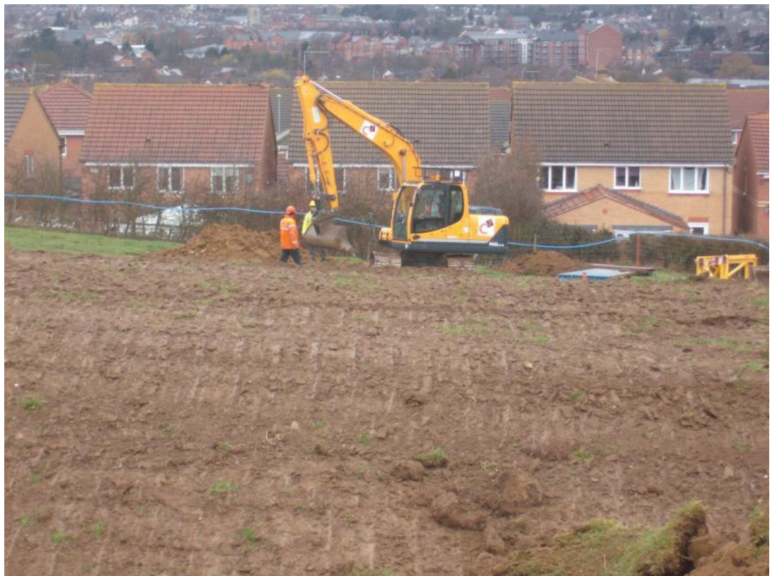
General view of the groundworks, looking west Fig 7
