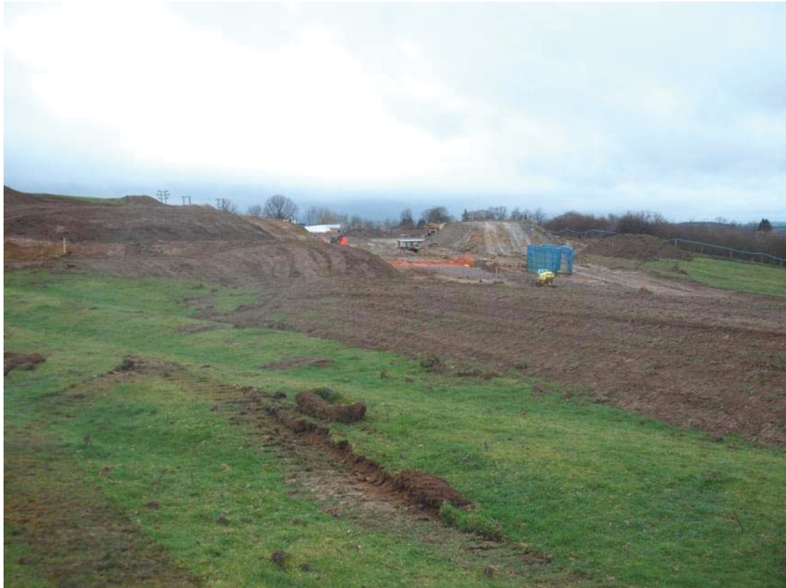
The investigation area, looking south Fig 4
