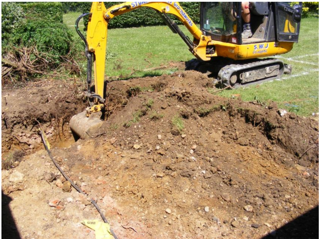
The groundworks in progress Fig 5
