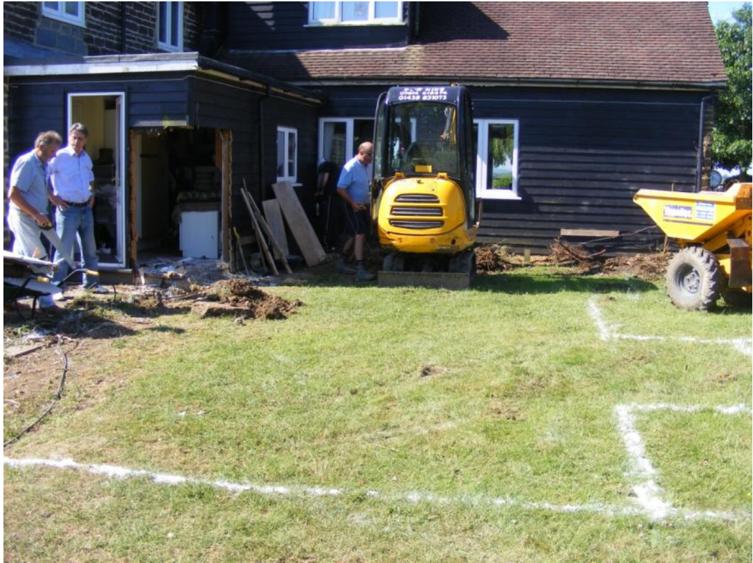
The development area at the start of groundworks Fig 4
