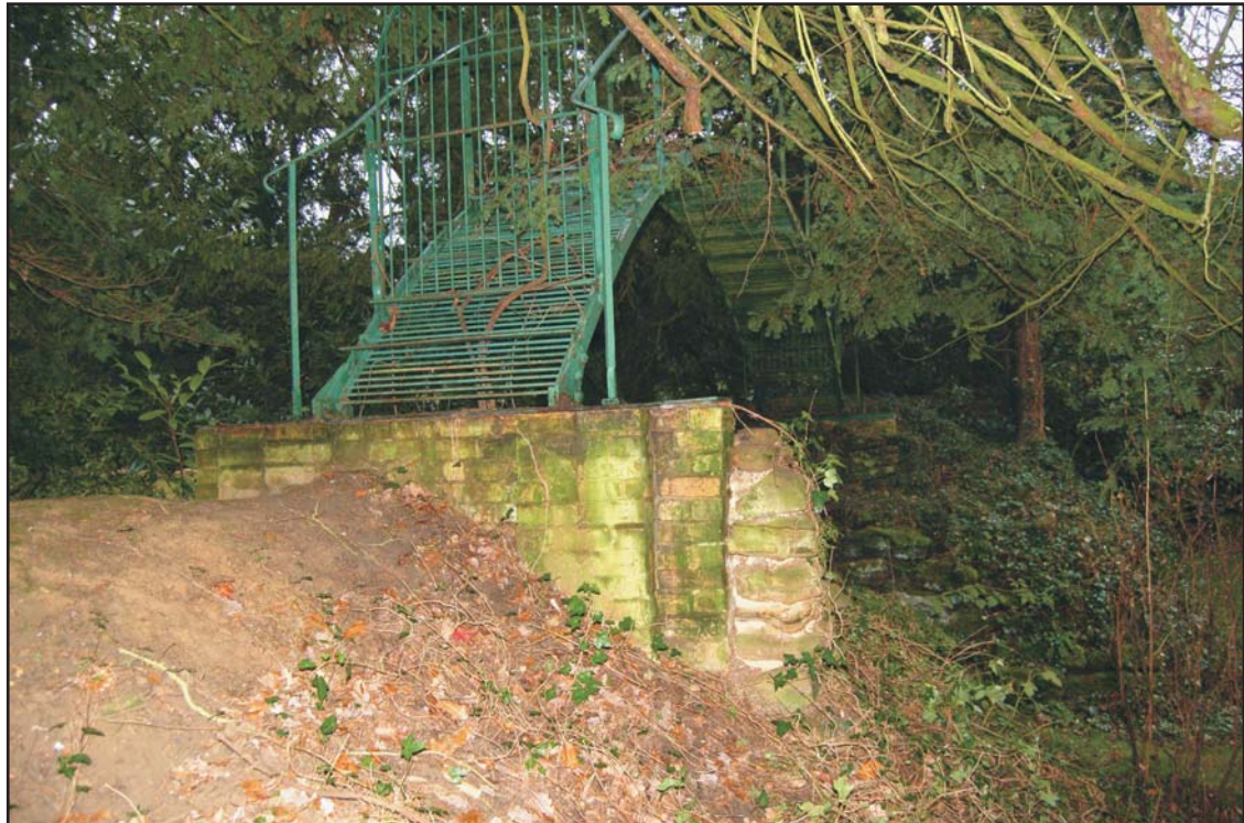
The Aerial Walkway showing the stone facing of the brick core, looking south Plate 10
