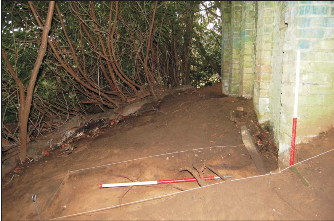
Trench Two, the eastern arm of the trench, looking south Plate 7
