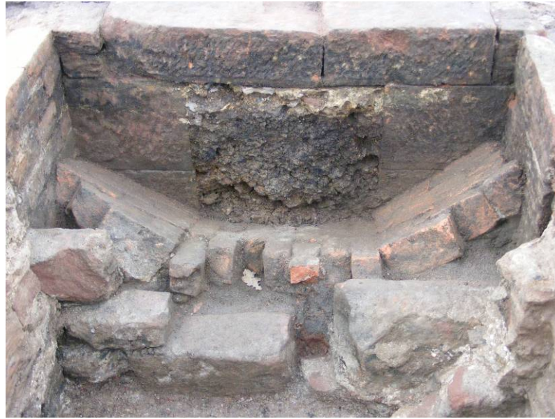
Chute on east side of agricultural trough Fig 14
