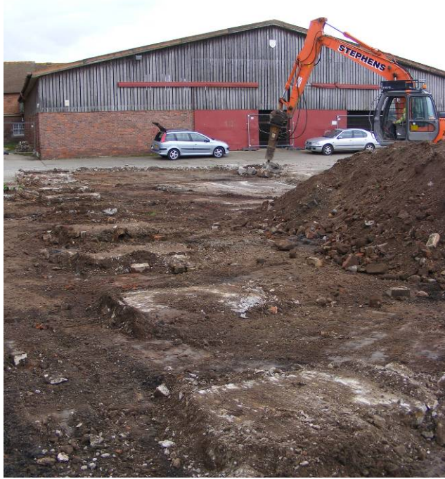
Breaking the concrete Fig 7
