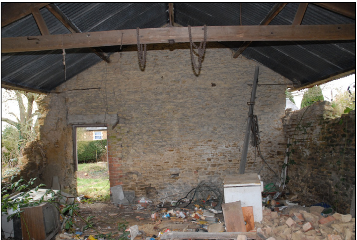
The eastern wall of Room 1 Fig 10
