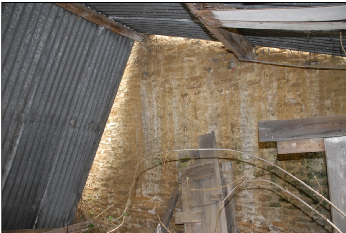
The eastern wall of Room 3 Fig 24
