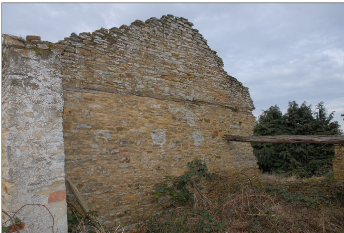
The western elevation, showing the timber course and extraneous timber Fig 16
