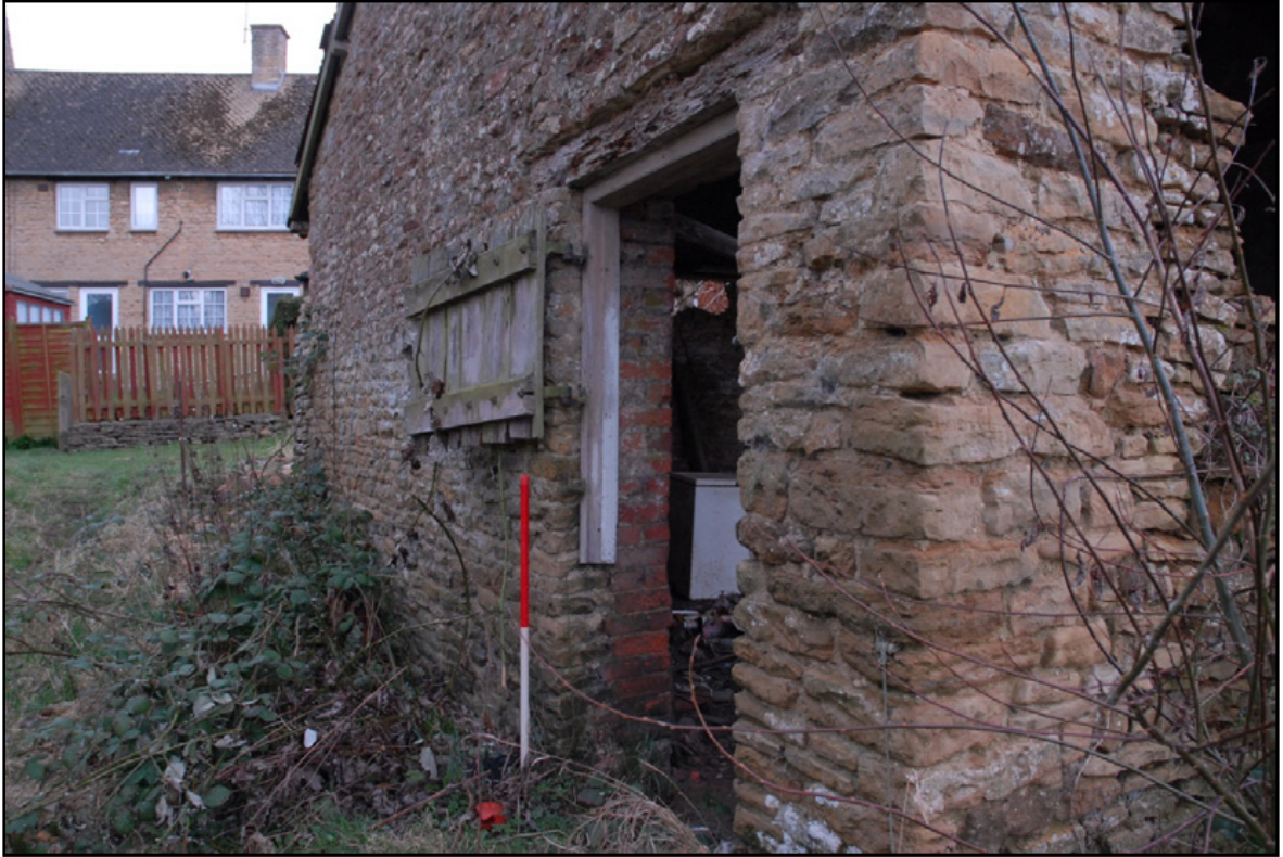
The doorway to Room 1, showing the internal brick jamb, looking south Fig 9
