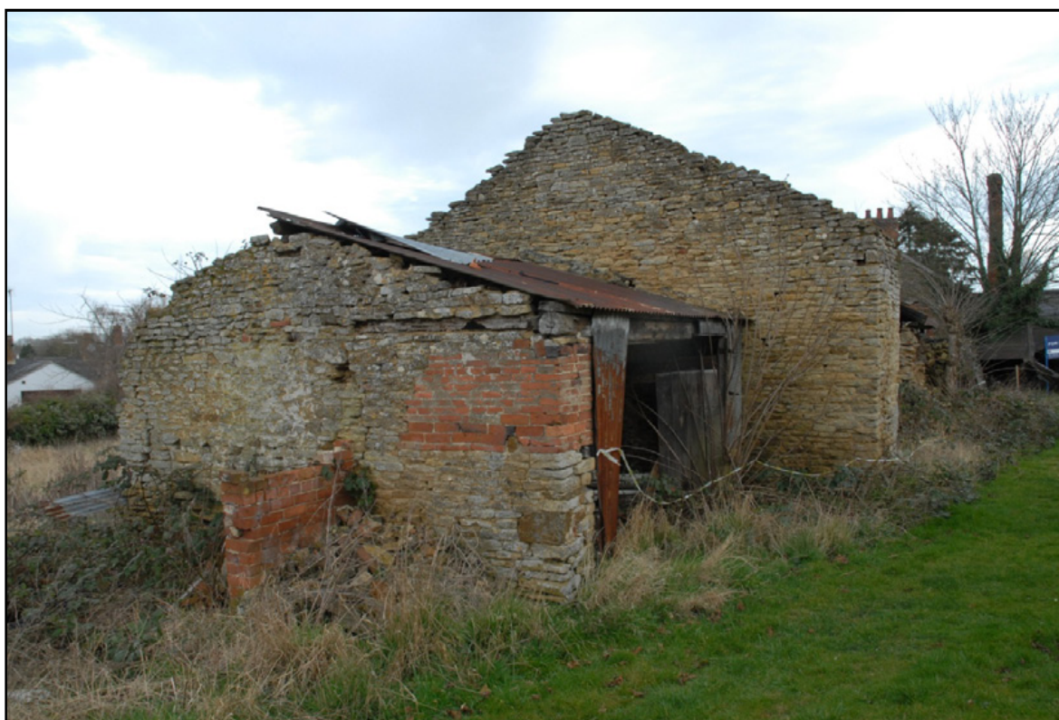
General view of the buildings, looking north-east Fig 4
