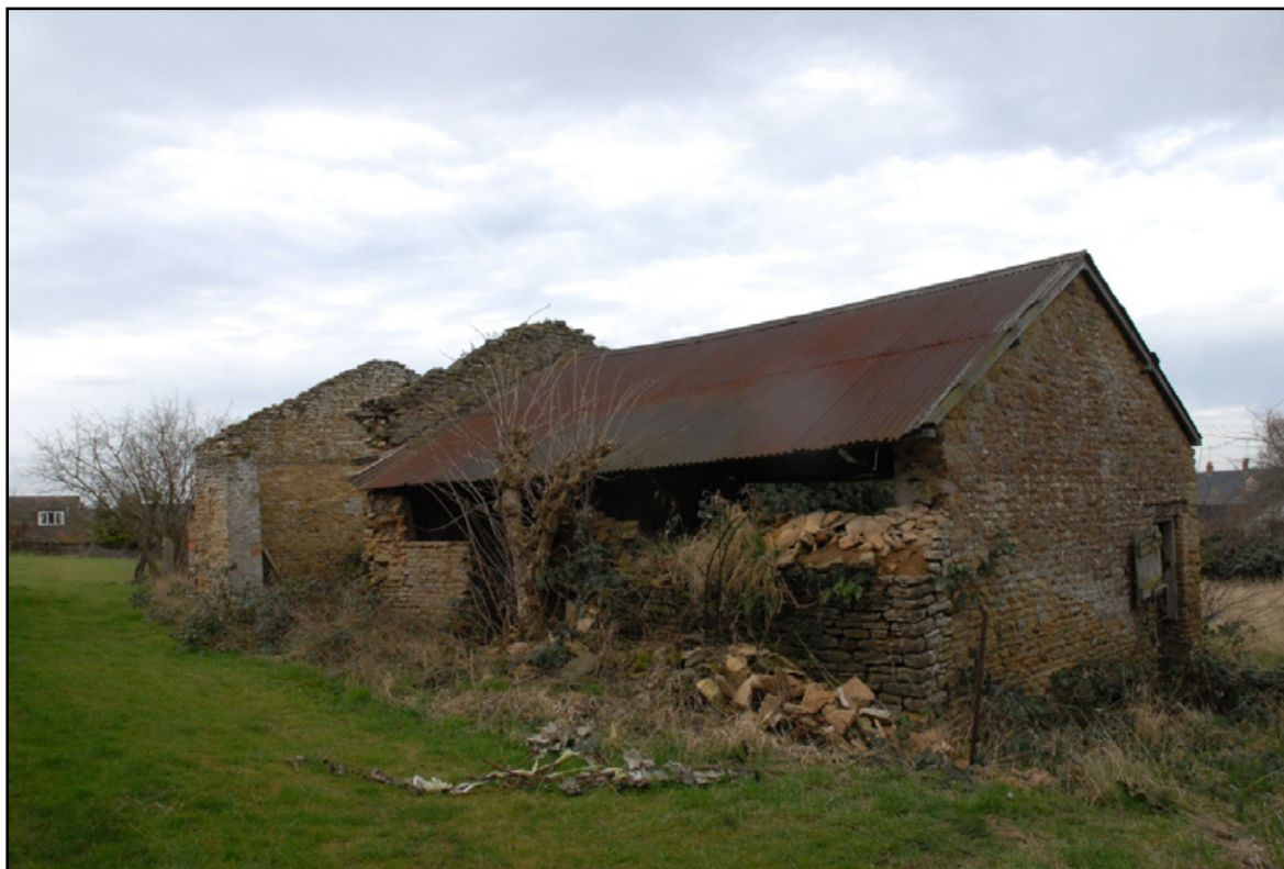
The southern elevation, looking west Fig 3
