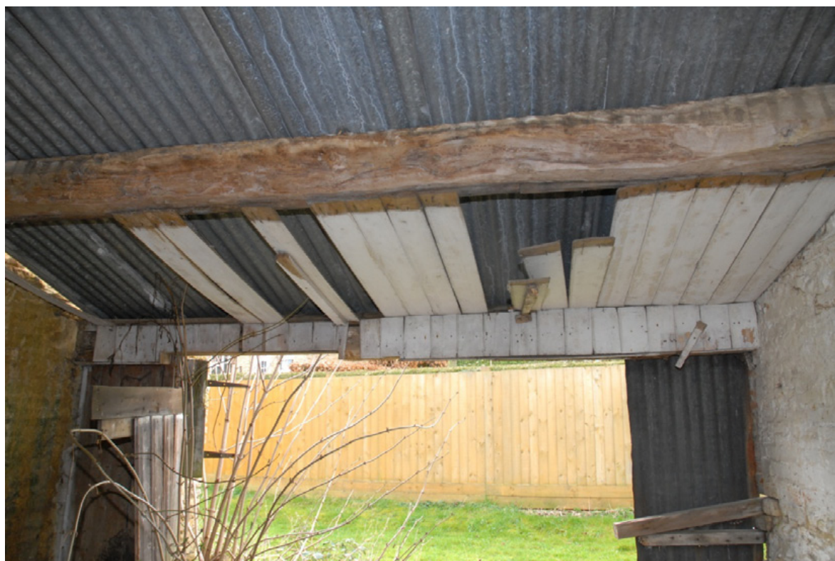
The white painted, wood cladding below the roof of Room 3 Fig 25
