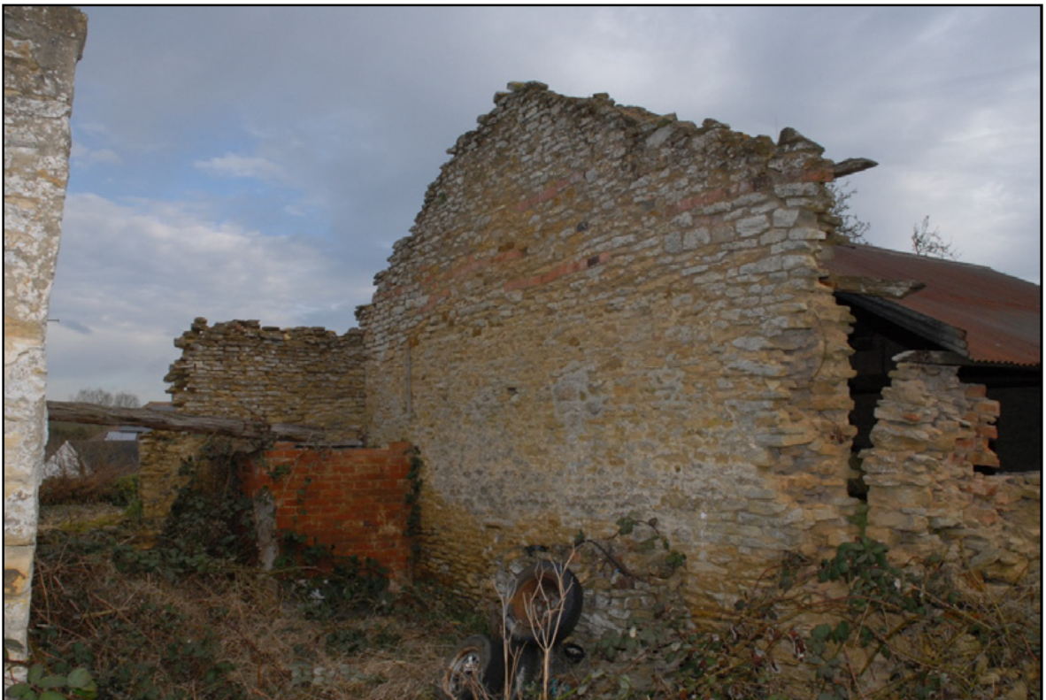
The eastern gable showing patches of red brick Fig 18
