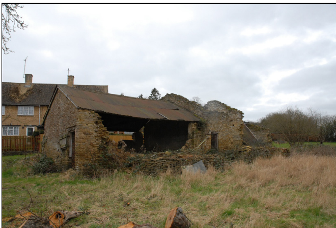
The northern elevation, looking south-west Fig 6
