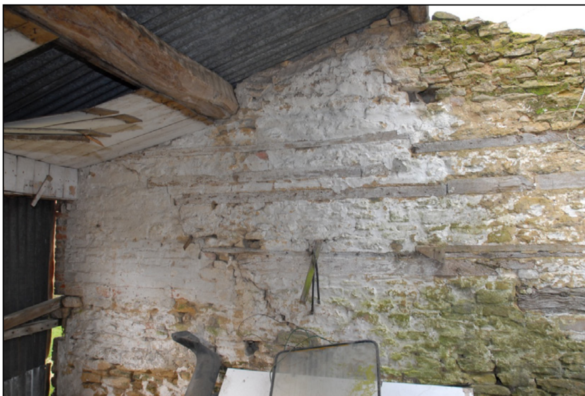
The western wall of Room 3 Fig 23
