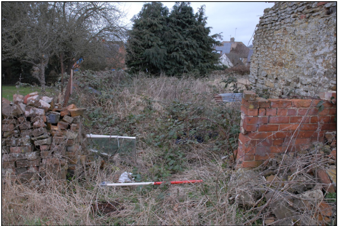
General view of Room 4 with the surviving brick wall to the right Fig 26
