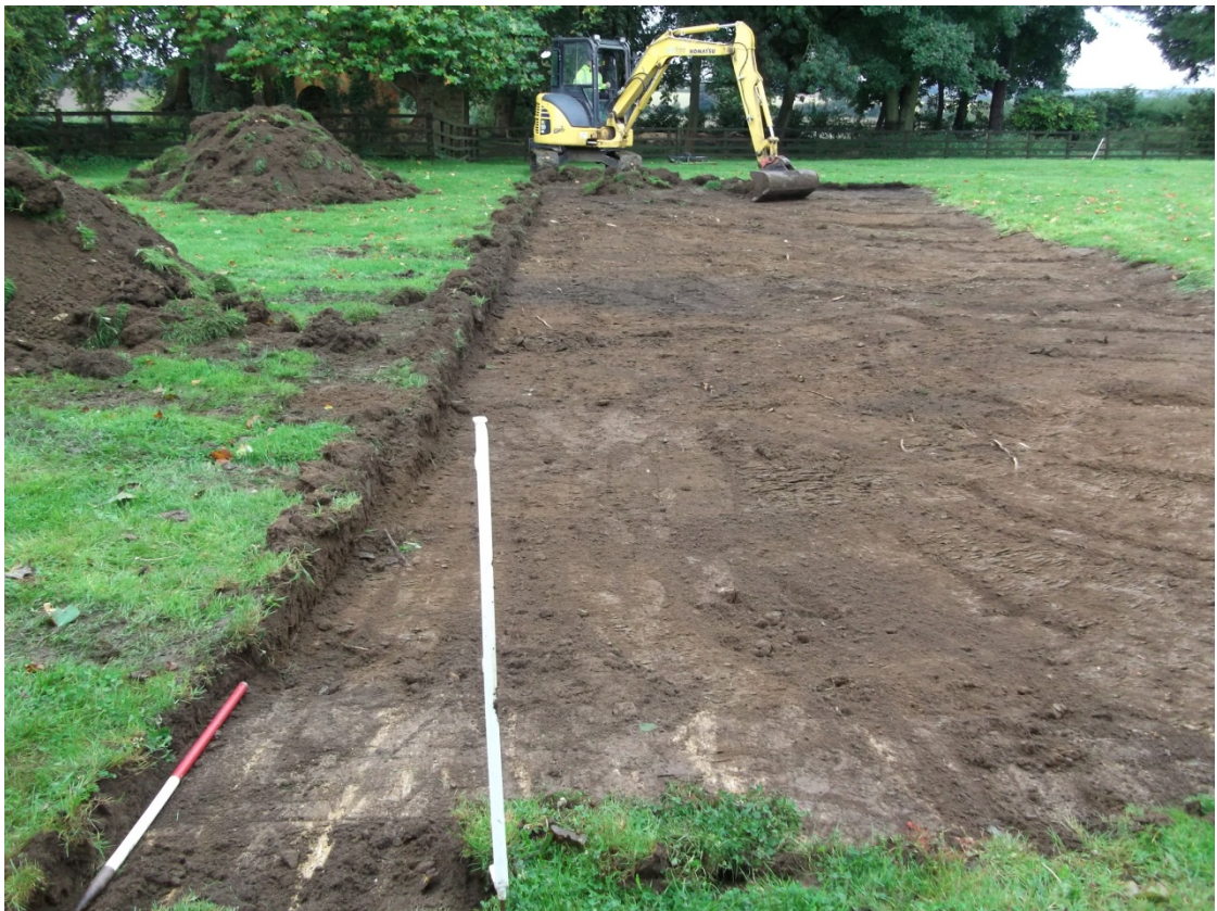
General view of the groundworks, looking west Fig 4
