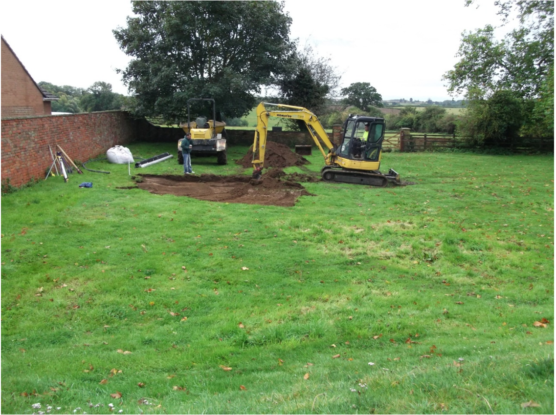
General view of the groundworks, looking south Fig 3
