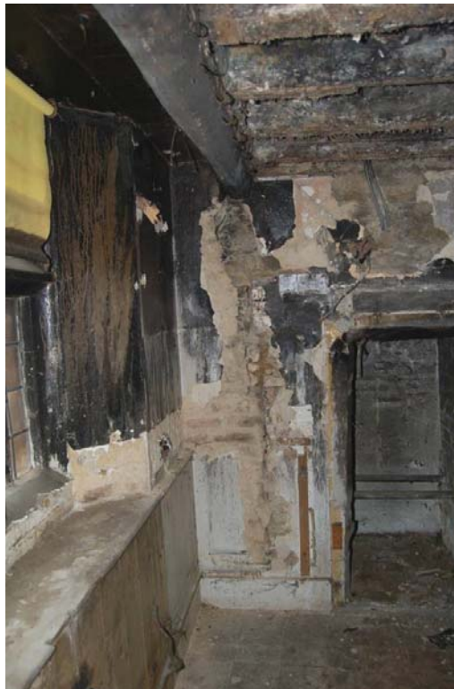
Room G4: moved west wall evidence Fig 13
