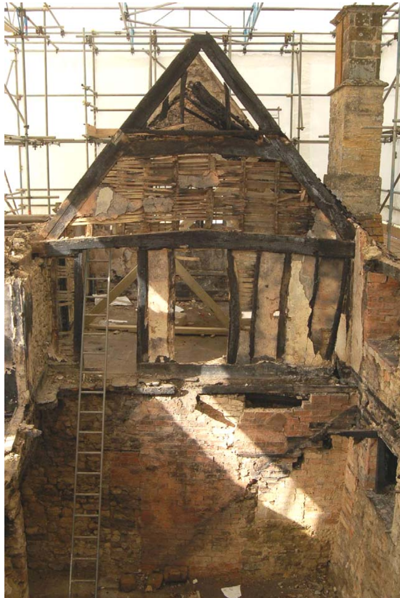
Room G2 (and F2), west wall and roof truss
