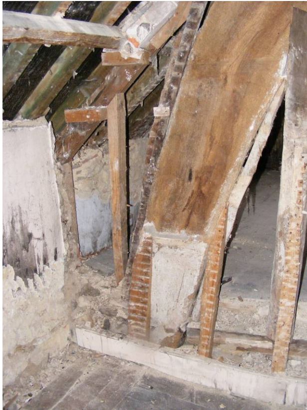
Cruck blade in south range (seen in Room F7) Fig 6
