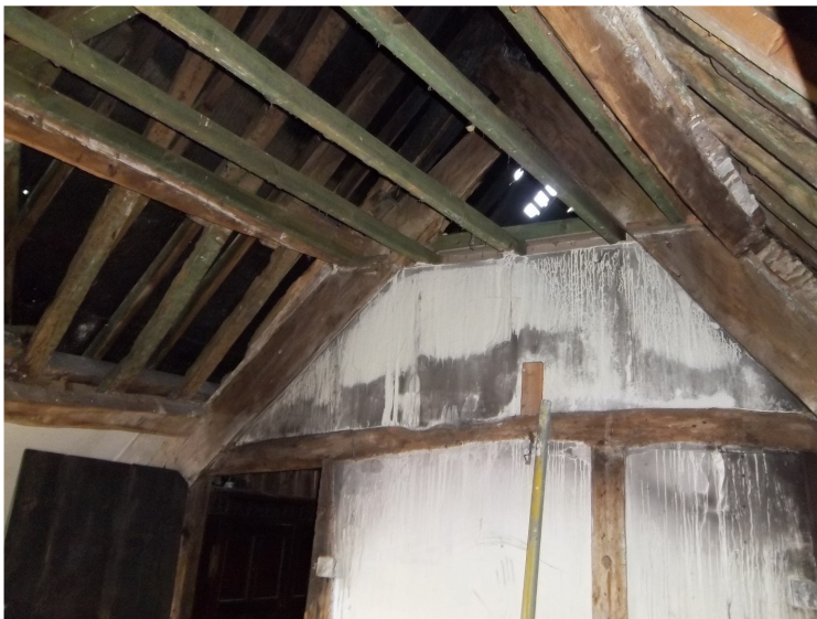
Figure 3d/e/f: Views of cruck truss in the south range (top and middle), and the principal rafter truss to the southern end of the south range roof
