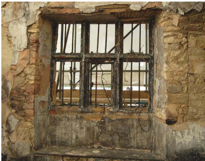
Room F1, west wall: evidence of former window Fig 11
