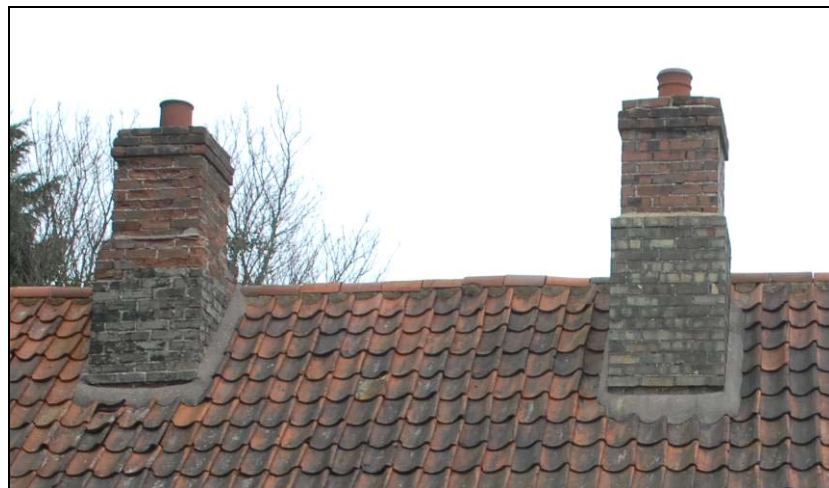
Chimney detail, looking east, showing the change in brickwork
