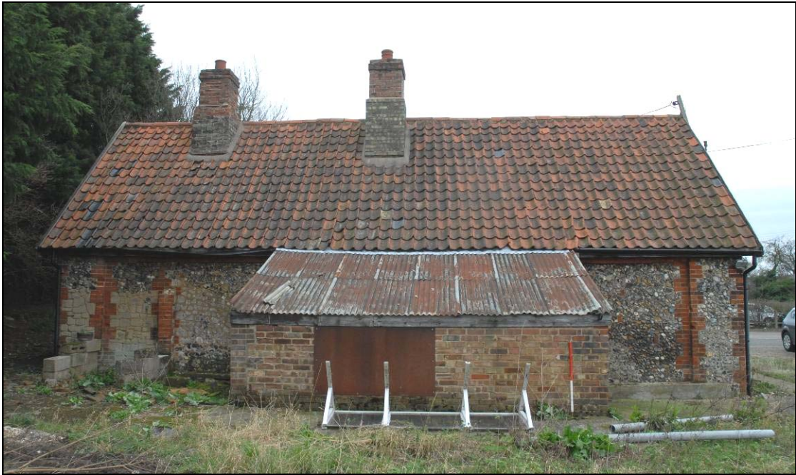
Rear elevation, looking east
