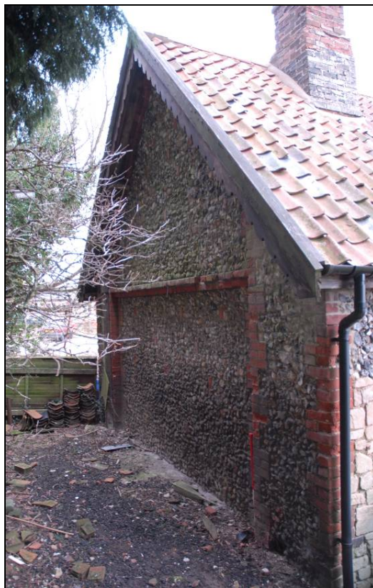
North gable end, looking south-east Fig 13
