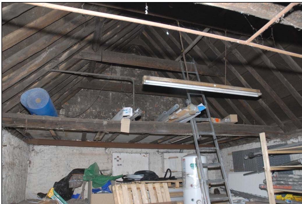
Open loft space at the southern end of the building Fig 18
