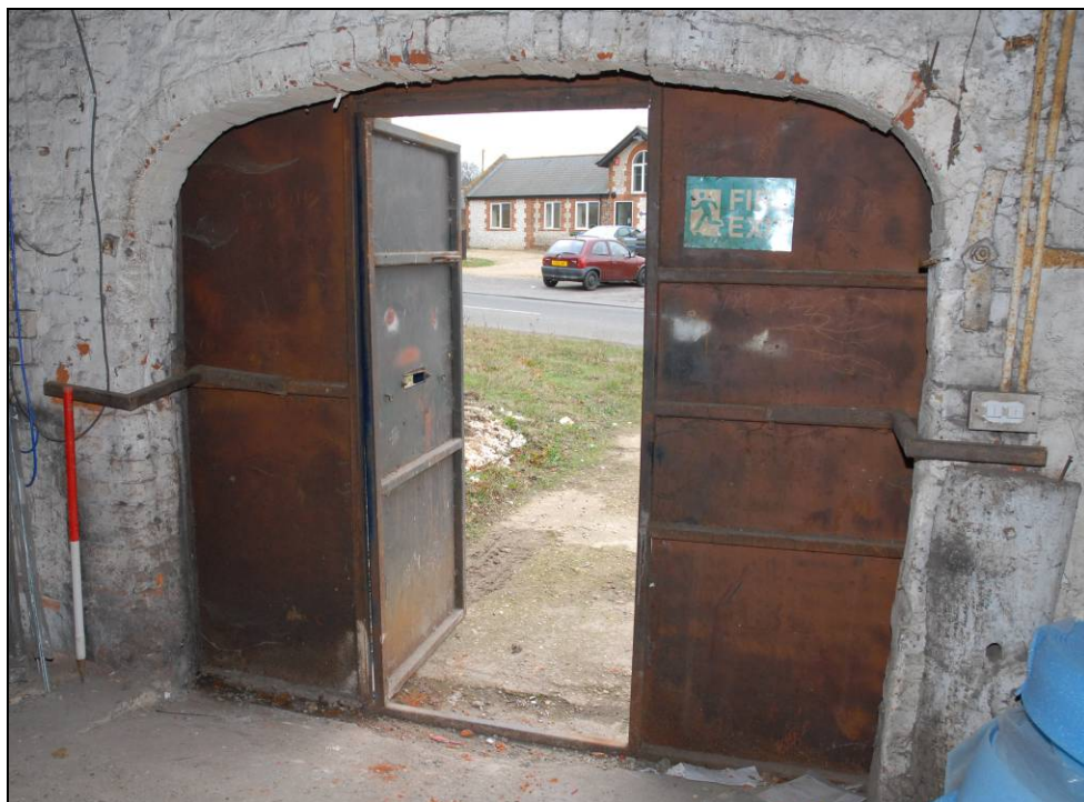
Main door into the forge showing the low brick arch over, looking east Fig 20
