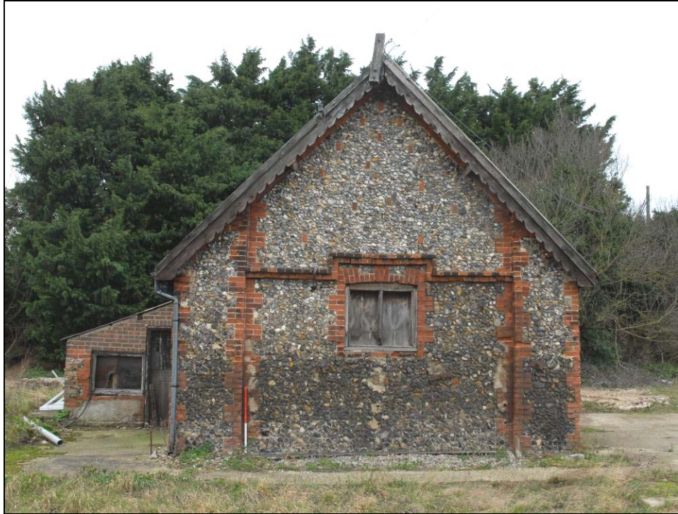
Gable elevation, looking north
