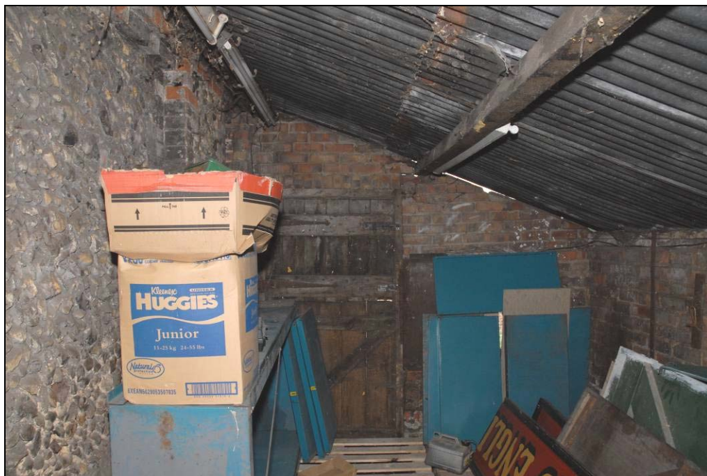
Interior of the lean-to looking south
