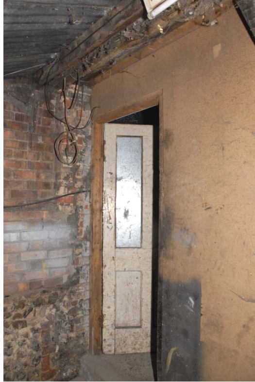
Interior of the lean-to showing the join, the door and the reduced opening Fig 22
