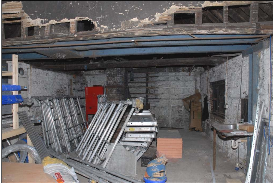
Forge interior, looking north, showing the lath and plaster partition at loft level Fig 14
