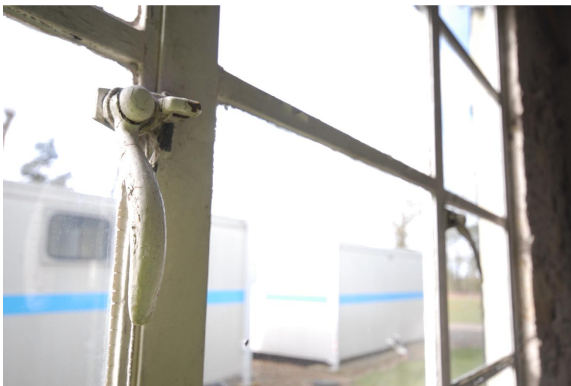
Building 2; original Crittall window with fittings
