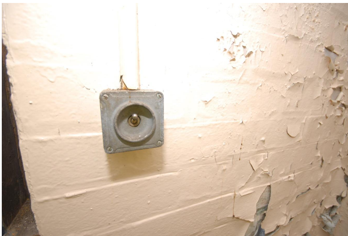
Building 13; original Bakelite switch
