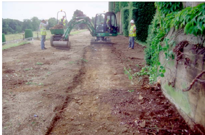
Plate 3 Stripping of scaffolding foundation trench – east side of house
