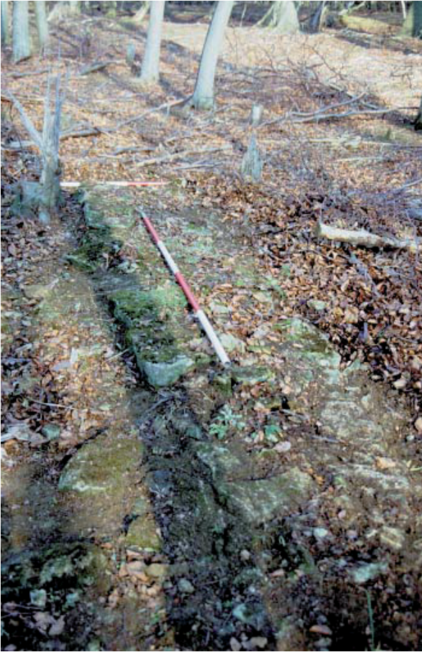
Plate 4: Site 1. Segment C. Wall 105, looking west.
