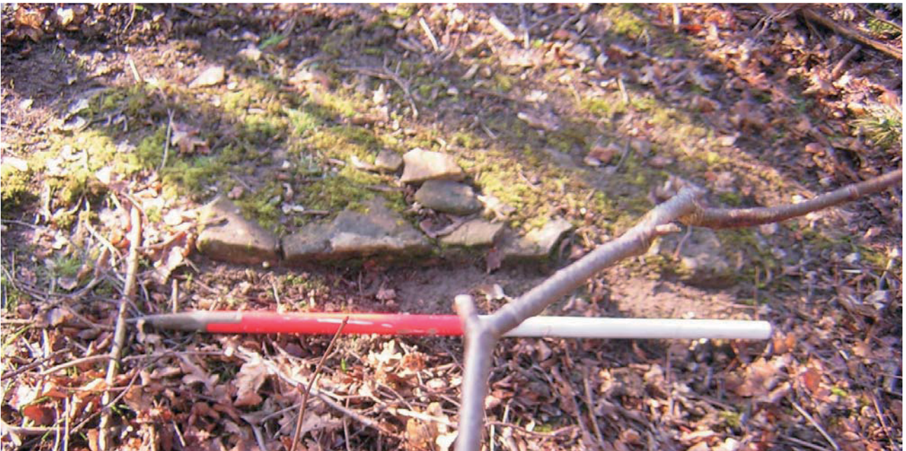
Plate 8: Site 2. Portion of Wall 201.
