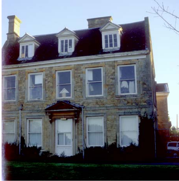
Plate 1 The west wing from the west
