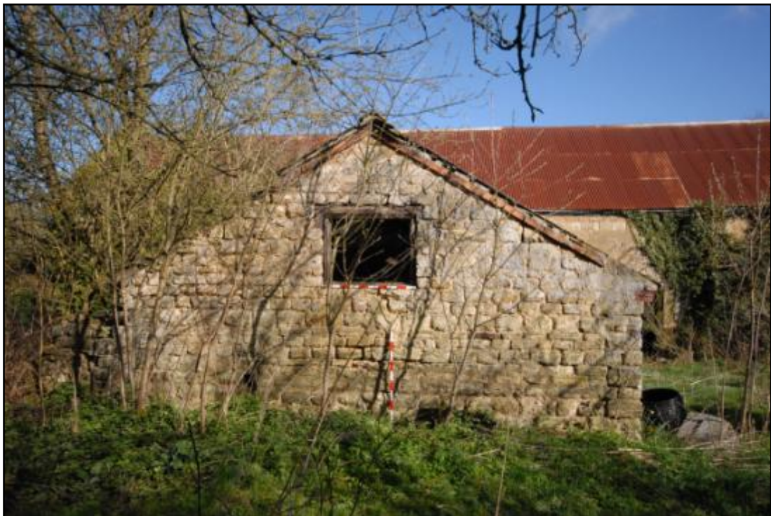
Stable 3, south elevation, looking north Fig 35
