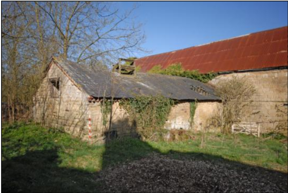
Stable 3, looking north-west Fig 34
