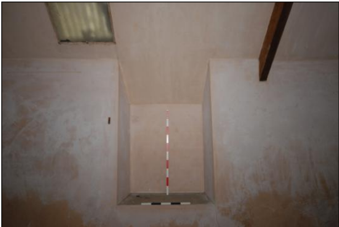
Detail of the Loft blocked window, looking north Fig 19
