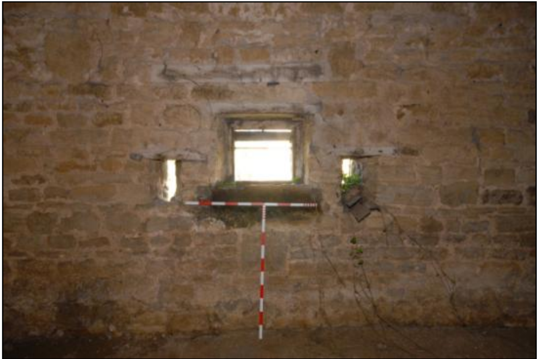
Detail of window in Crop Barn Fig 32
