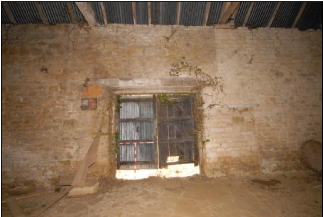
The reduced door, showing blockings, looking south Fig 29
