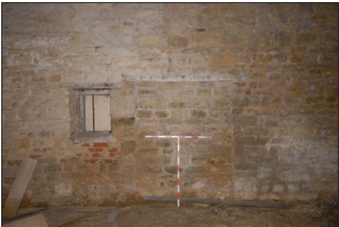
Detail of blocked door Fig 33
