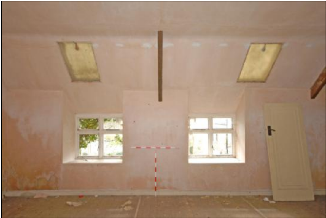
South wall of the Loft, looking south Fig 18
