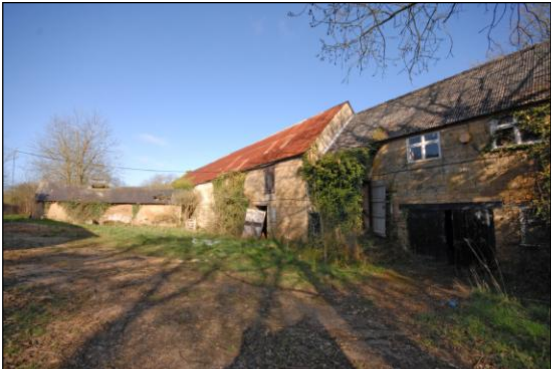
General view of the buildings, looking west Fig 4
