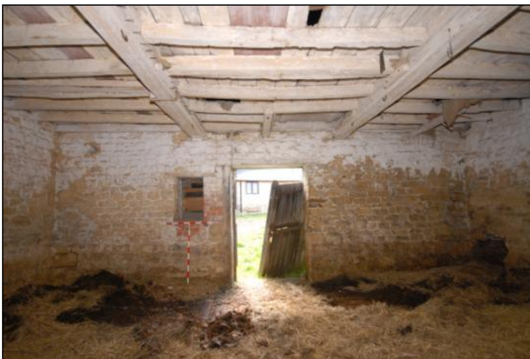
Stable 1, interior, looking south Fig 21
