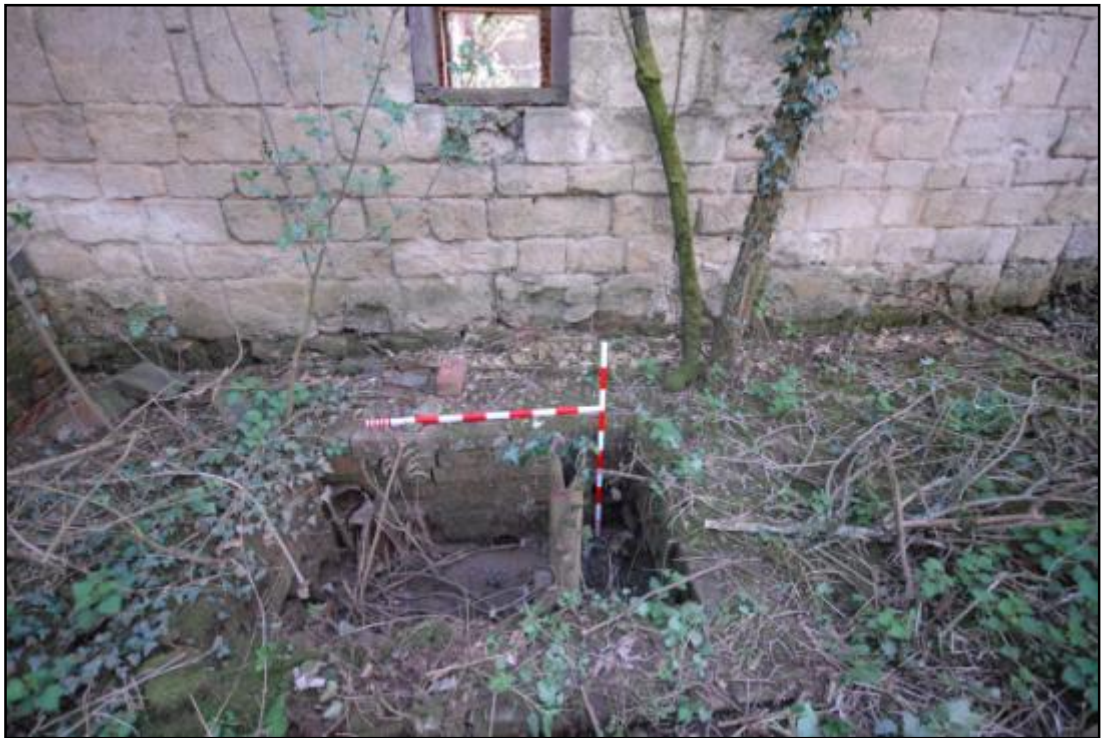
The sump to the west of the Lean-to, looking south Fig 45
