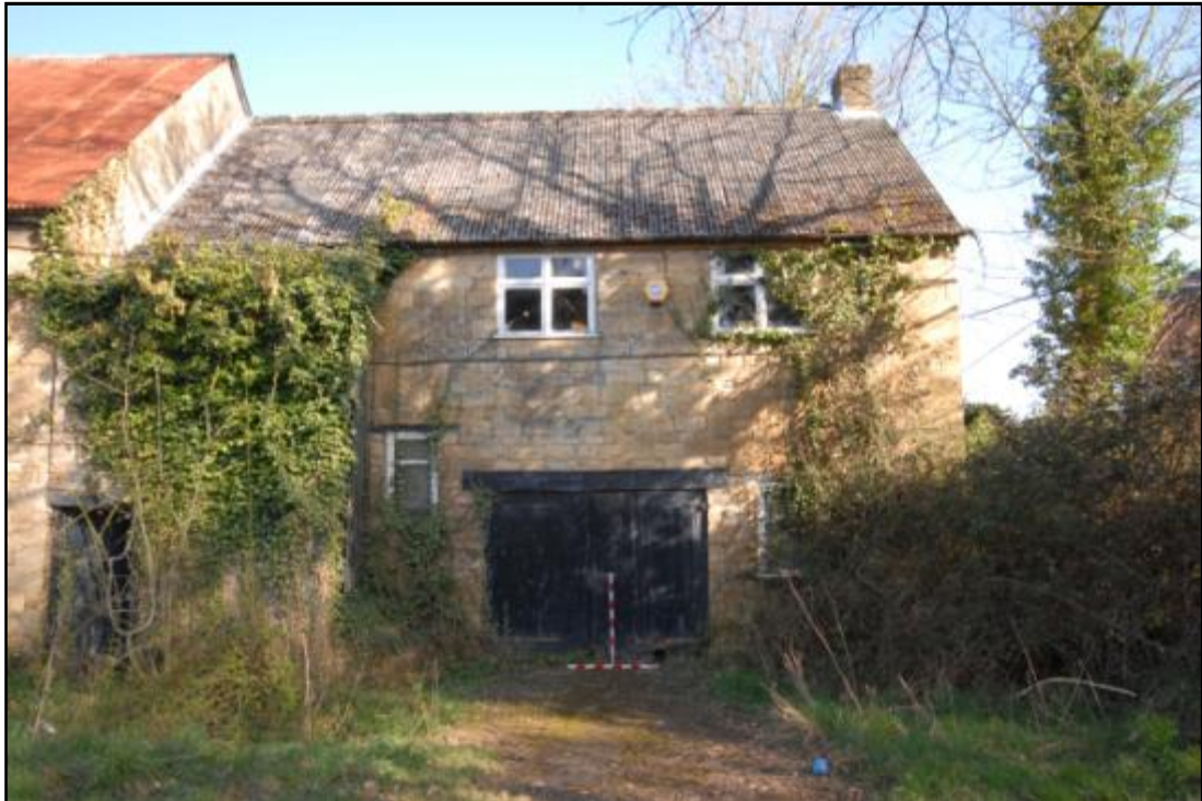
Harness Room and Loft, south elevation, looking north Fig 11
