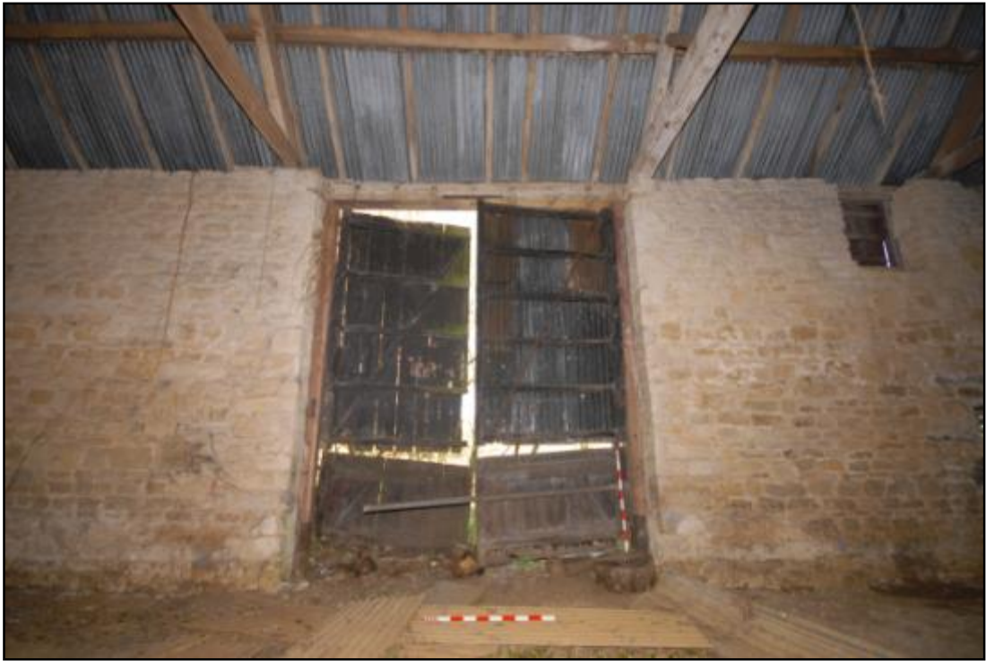
The north opening Crop Barn door, looking north Fig 28
