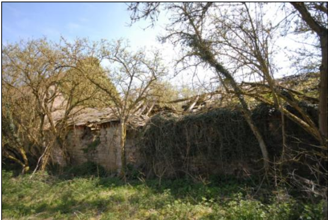
General view of the site, showing Stable 4, looking south-east Fig 8
