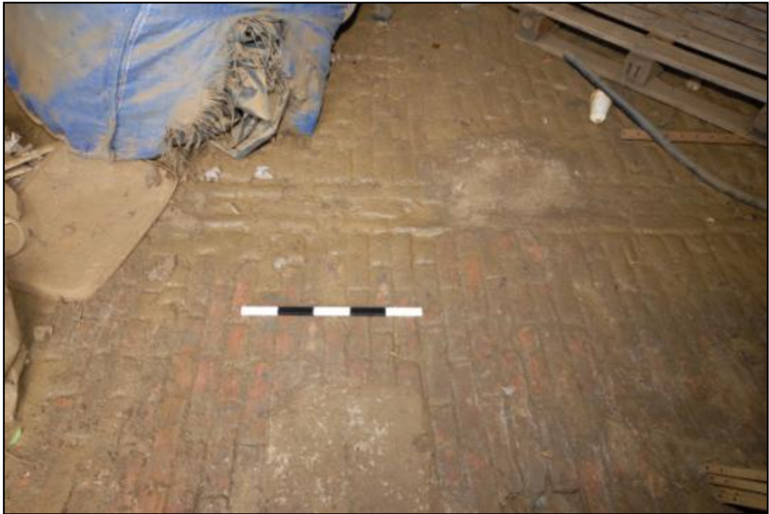
Detail of the Harness Room floor showing brick drain Fig 14
