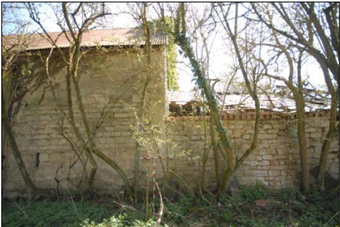
Stable 4, north elevation, showing join with Crop Barn, looking south Fig 39
