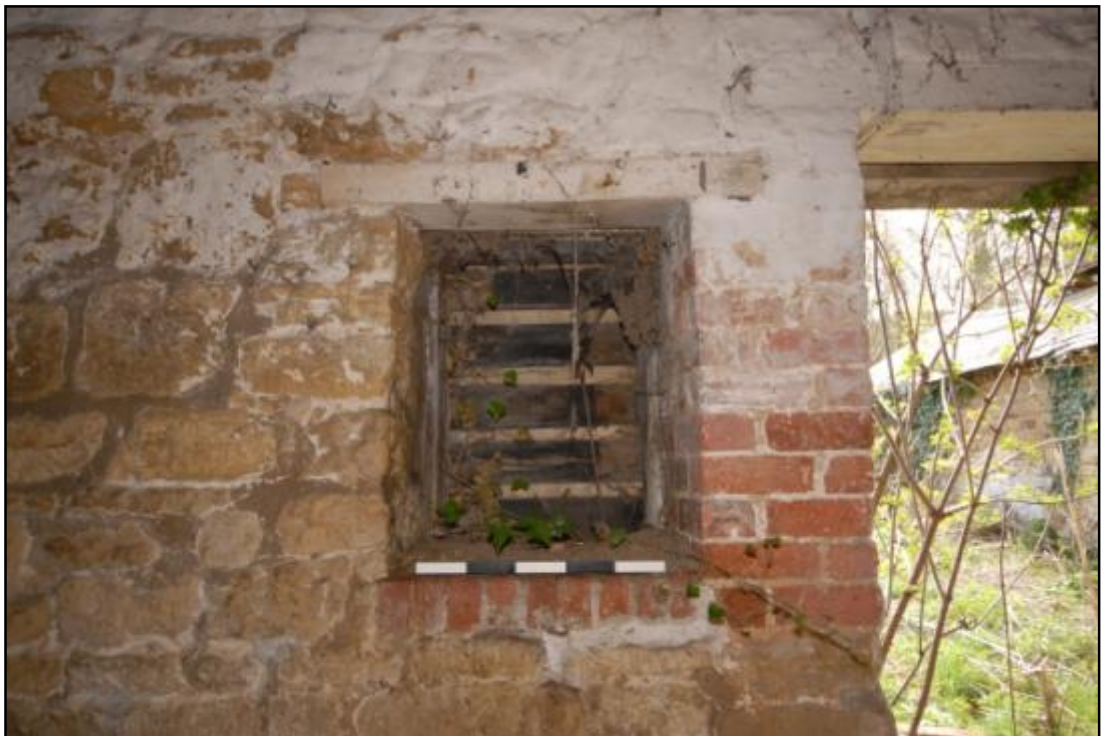
Detail of louvered window in Stable 2 Fig 25
