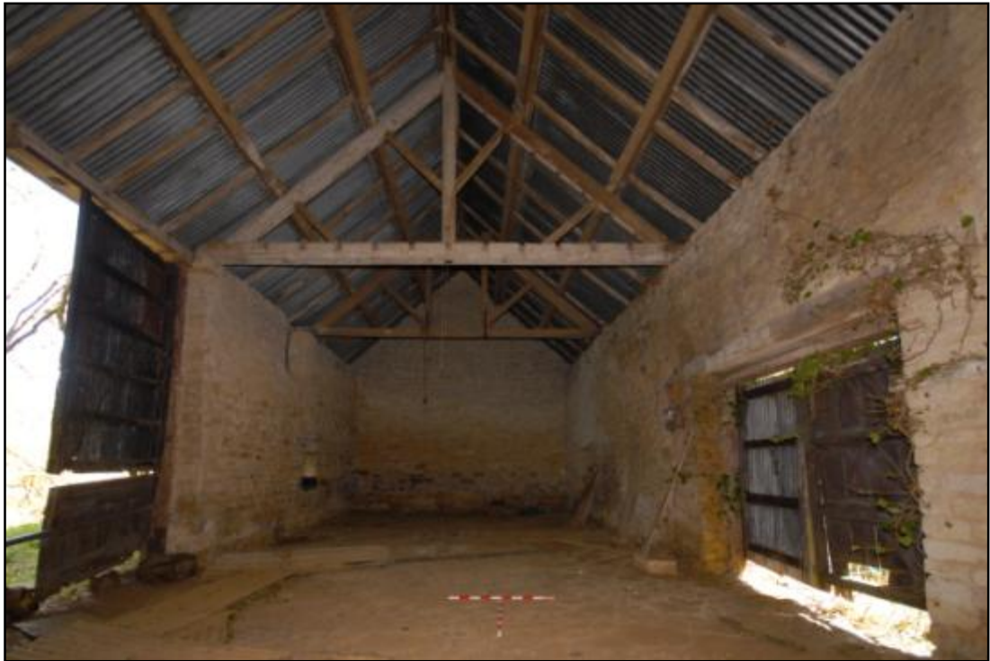
Crop Barn, interior, looking east (note reused timber in truss) Fig 30
