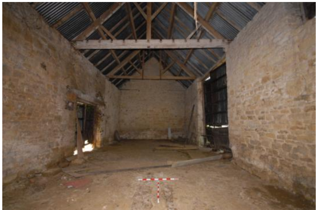
Crop Barn, interior, looking west Fig 31
