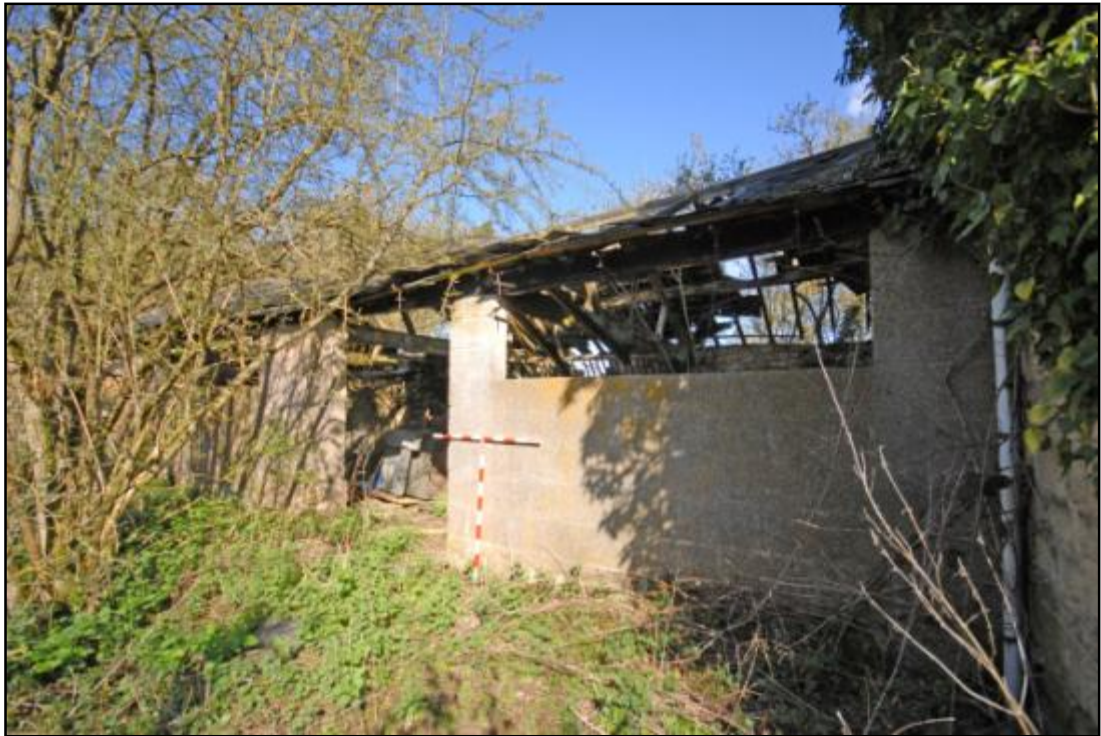
Stable 4, south elevation, looking north-west Fig 38
