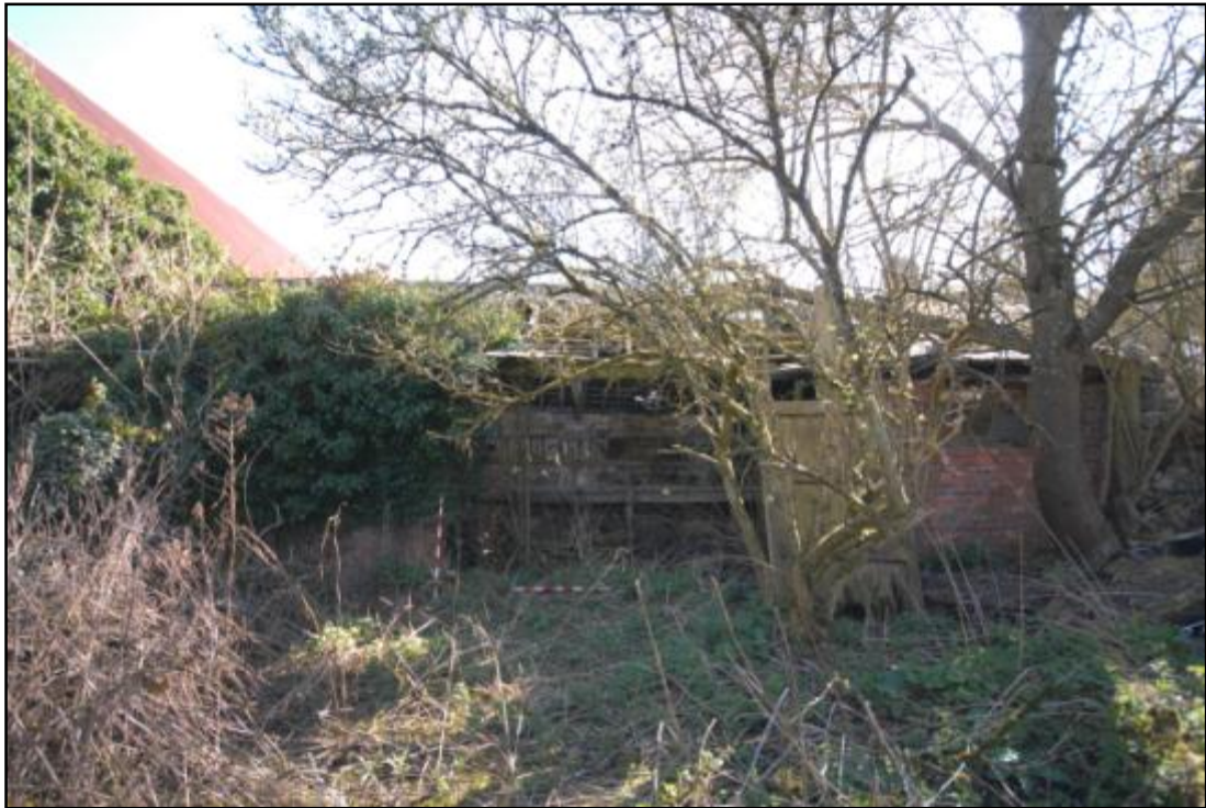
Stable 3, west elevation, looking east Fig 36
