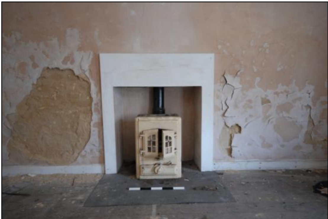
Detail of the fireplace and range Fig 17
