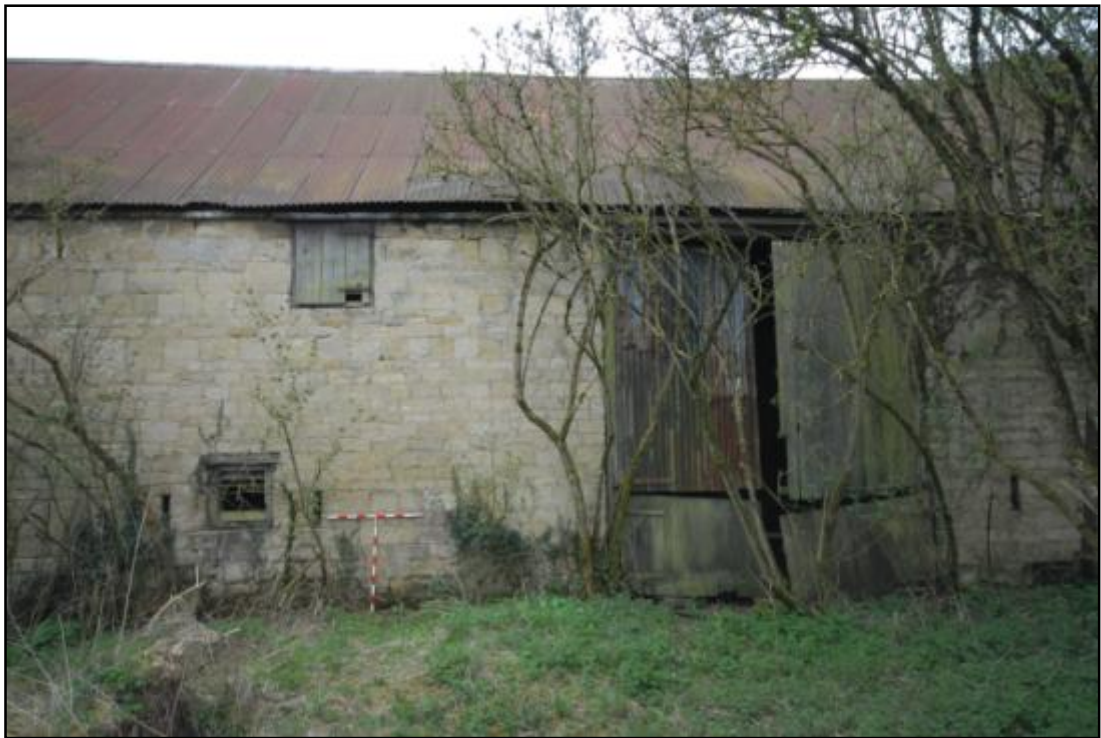
North elevation of the Crop Barn, looking south Fig 27
