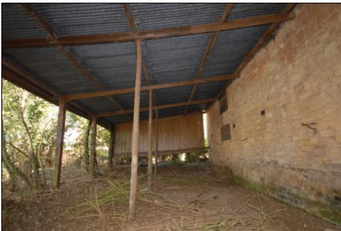
Lean-to, interior, looking east Fig 42
