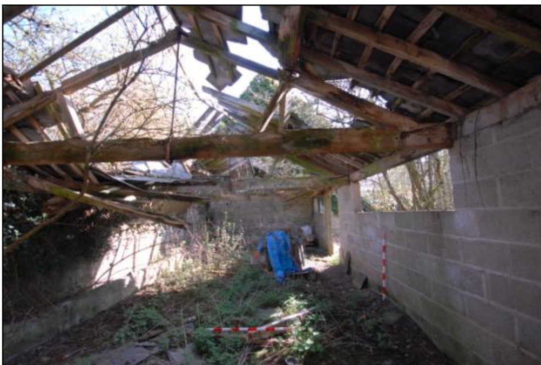
Stable 4, interior, looking east Fig 41
