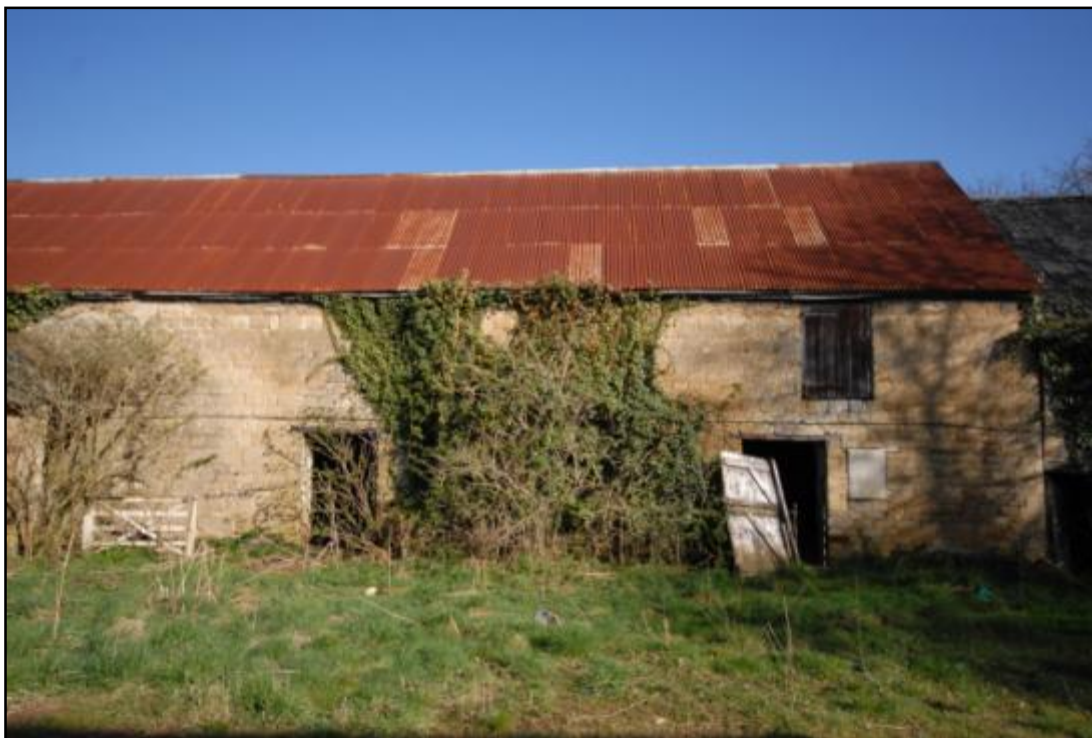
South elevation, Stable 1 and Stable 2, looking north Fig 20
