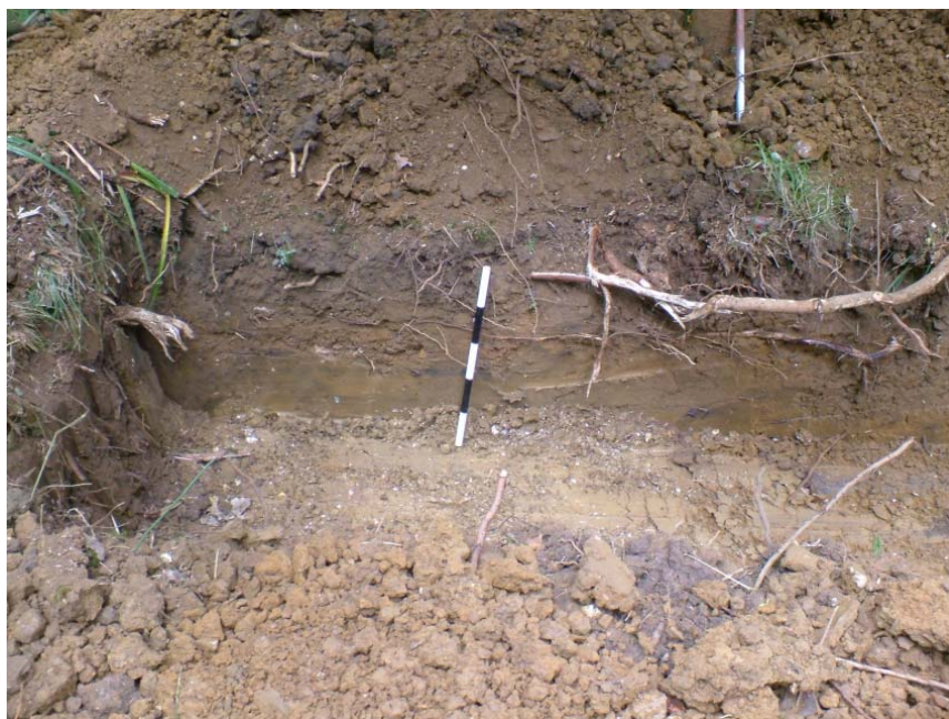
Plate 1: Foundation for Tower 13
