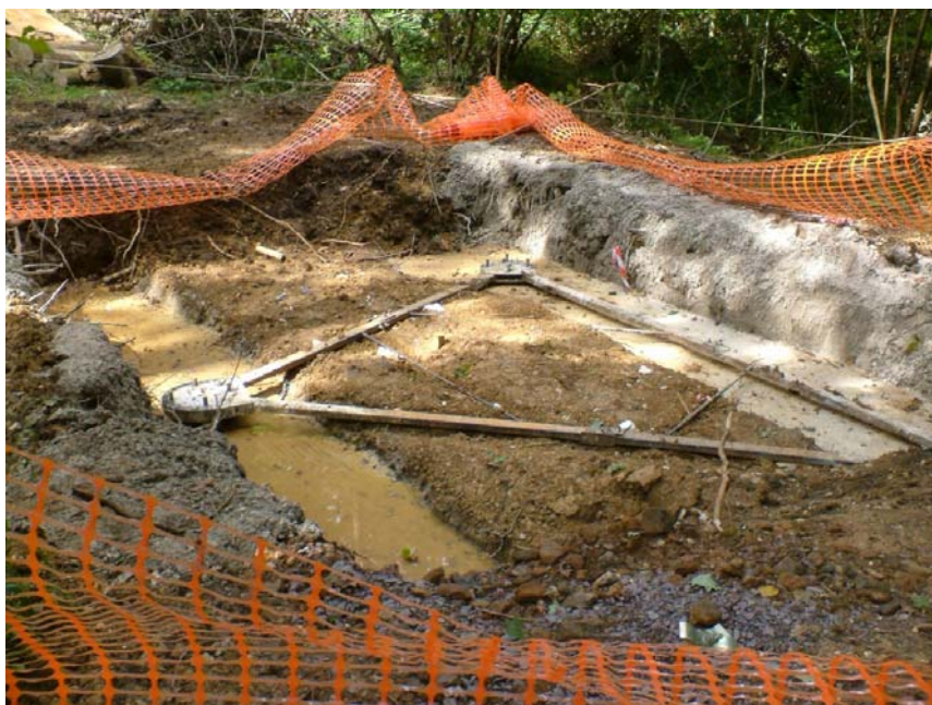
Plate 2: Steel base for tower concreted in, Tower 13
