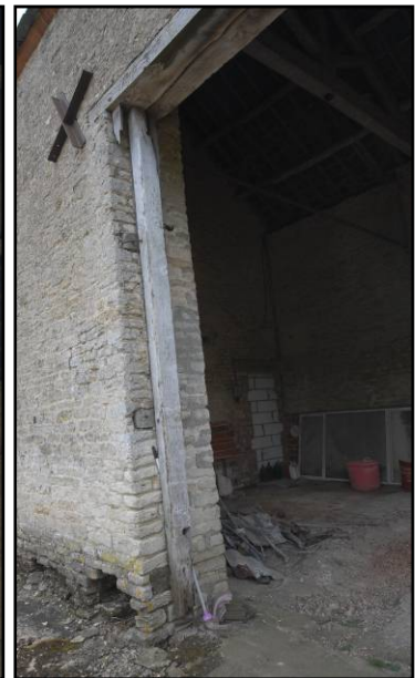
Door jamb, looking east Fig 21
