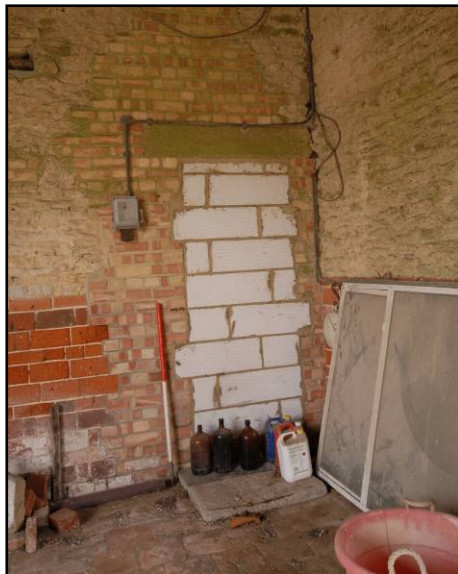
North-eastern door, Fig 23 looking north-east
