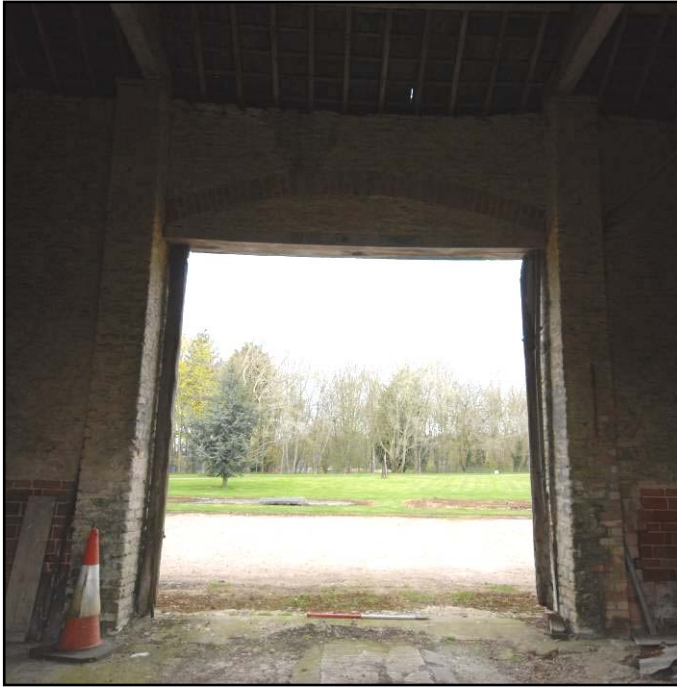
Stone pilasters, looking north-west Fig 18
