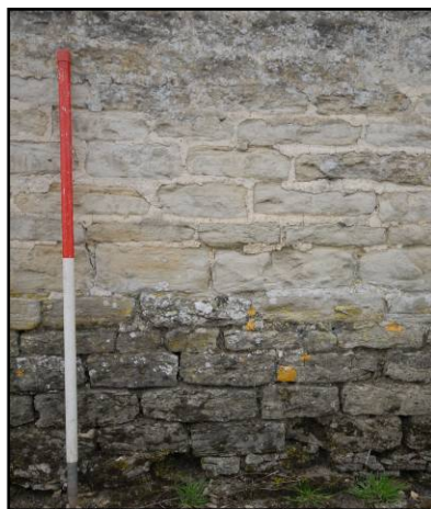
External limestone wall, Fig 14 looking north-west
