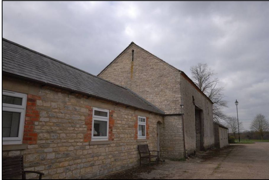
Side elevation, looking south-west Fig 7
