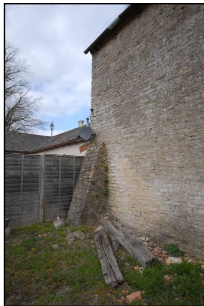
Buttress, looking north-west Fig 17
