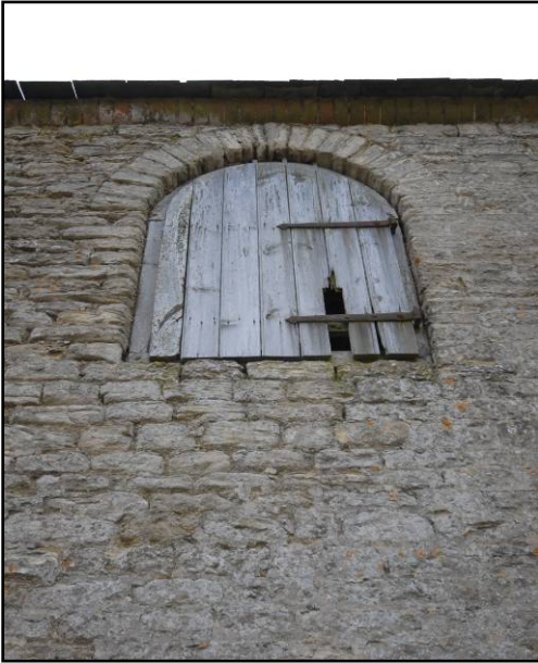
External view of window, Fig 25 looking south-east
