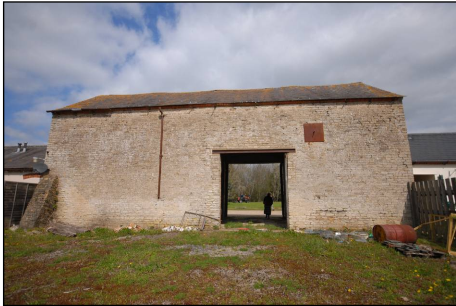
Rear elevation, looking north-east Fig 5
