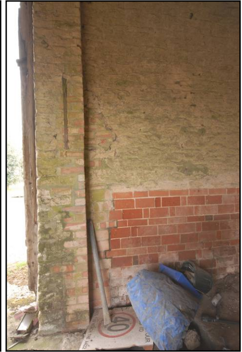
Brick repairs to pilaster, looking north-west Fig 19
