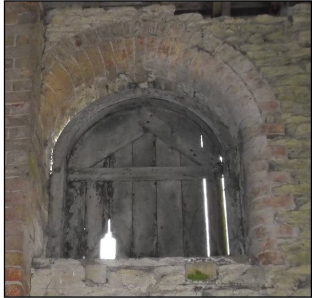
Internal view of window, Fig 26 looking north-west
