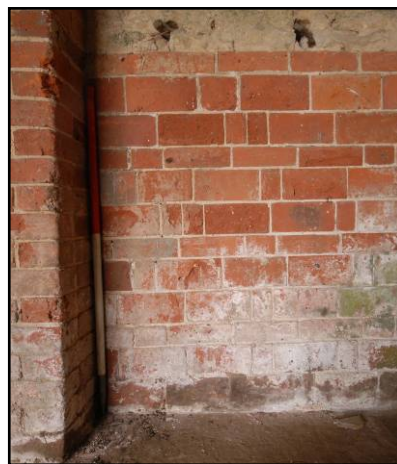
Internal brick wall, Fig 15 looking south-west
