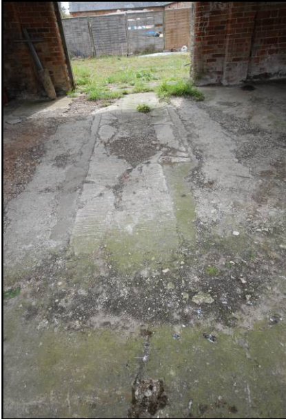
Central concrete area, Fig 29 looking south-east
