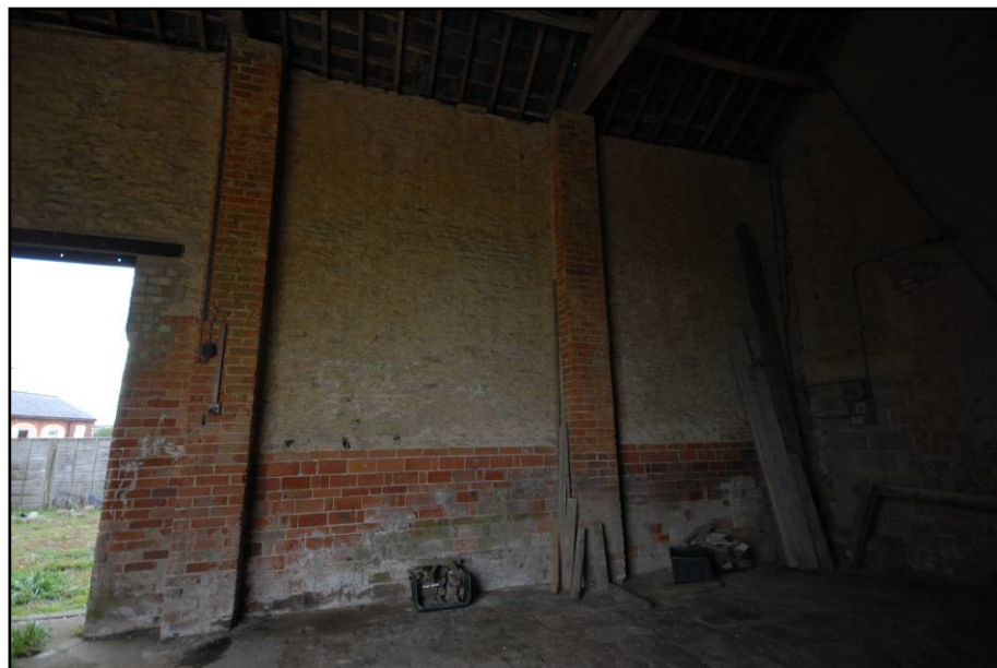
Right internal elevation beside rear barn door, looking south-east Fig 12
