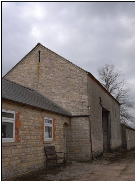
External view of window, Fig 27 looking south-west
