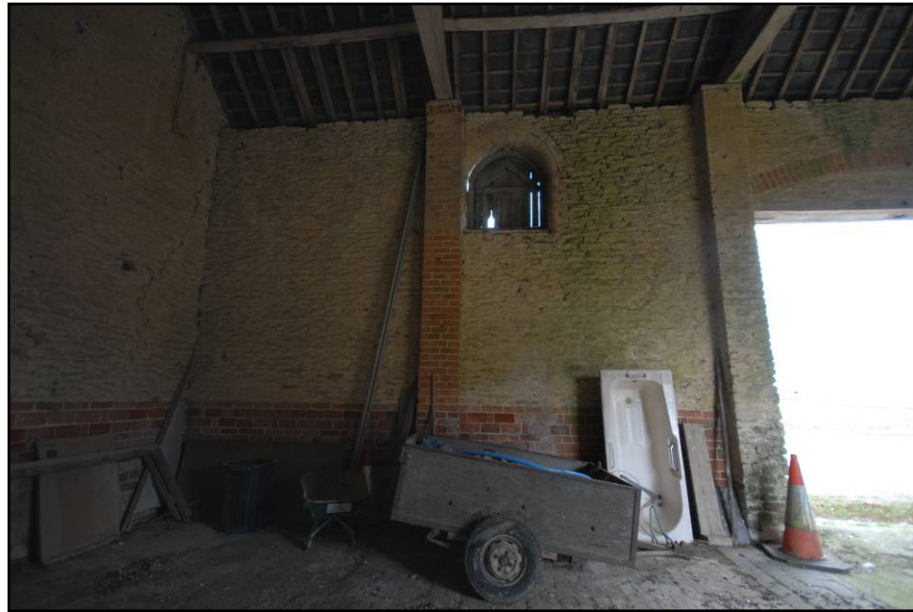
Left internal elevation beside front barn door, looking north-west Fig 9
