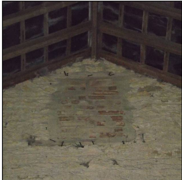
Internal view of window, Fig 28 looking south-west
