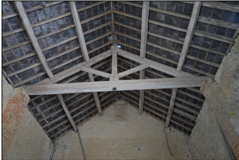
Machine sawn king post trusses, purlins, rafters and battens Fig 16
