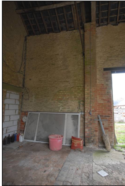
Right internal elevation beside rear barn door, looking south-east Fig 13
