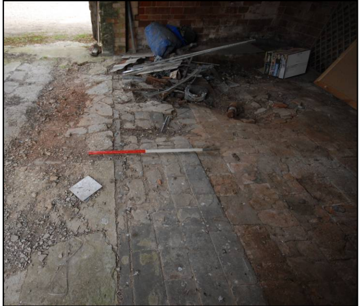
Blue brick border, looking north-west Fig 30
