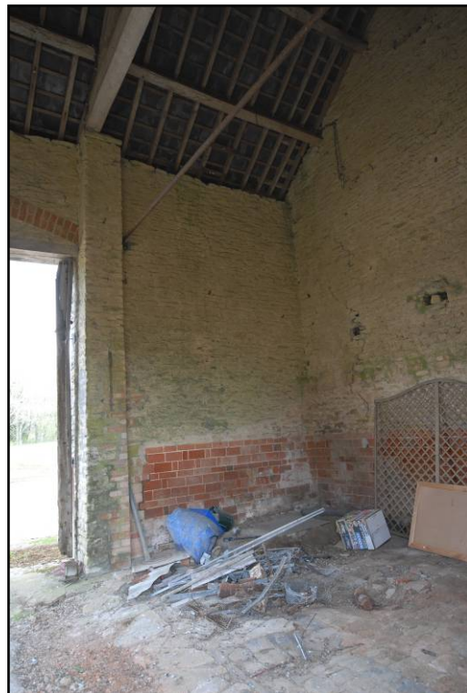
Right internal elevation beside front barn door, looking north-west Fig 10
