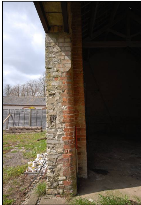
Original features and changes to door, looking south-west Fig 22
