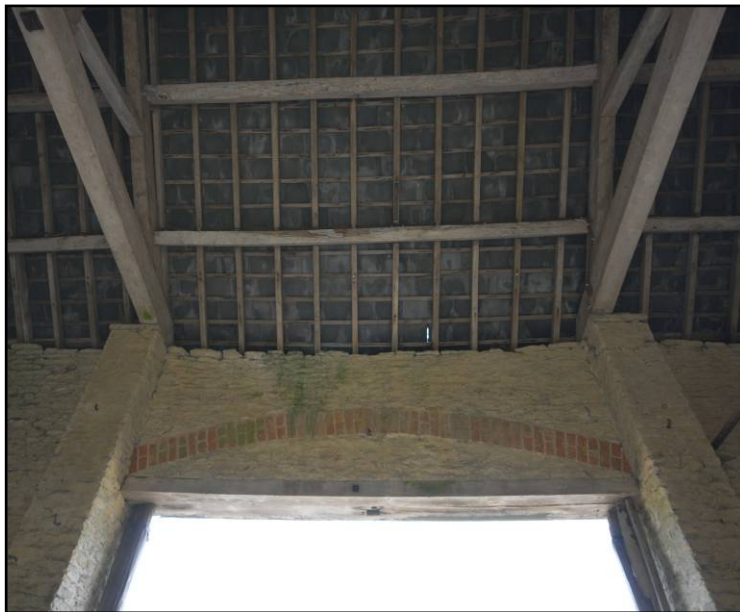
Brick segmental relieving arch, looking north-west Fig 20
