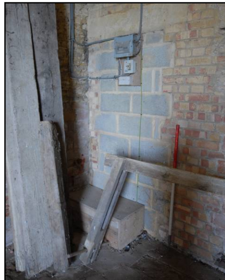
North-western door, Fig 24 looking north-west
