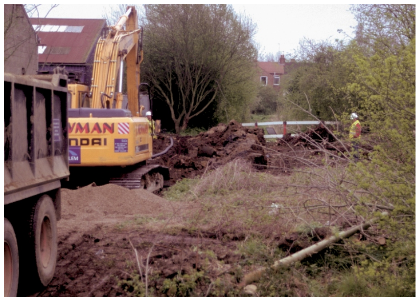
Plate 2: Working shot in area of Trench 6
