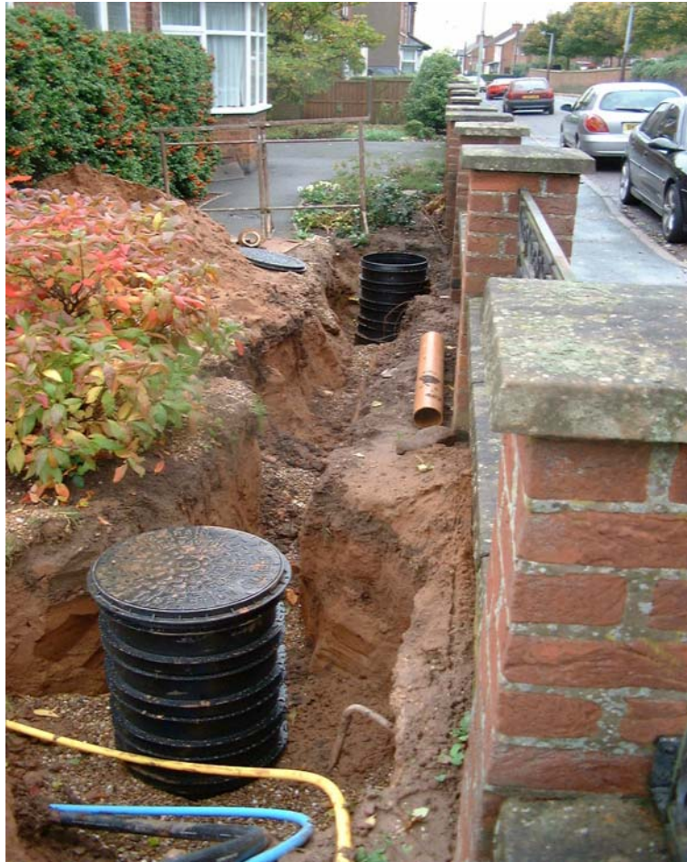
Plate 3: The drainage trench along the frontage of the development area
