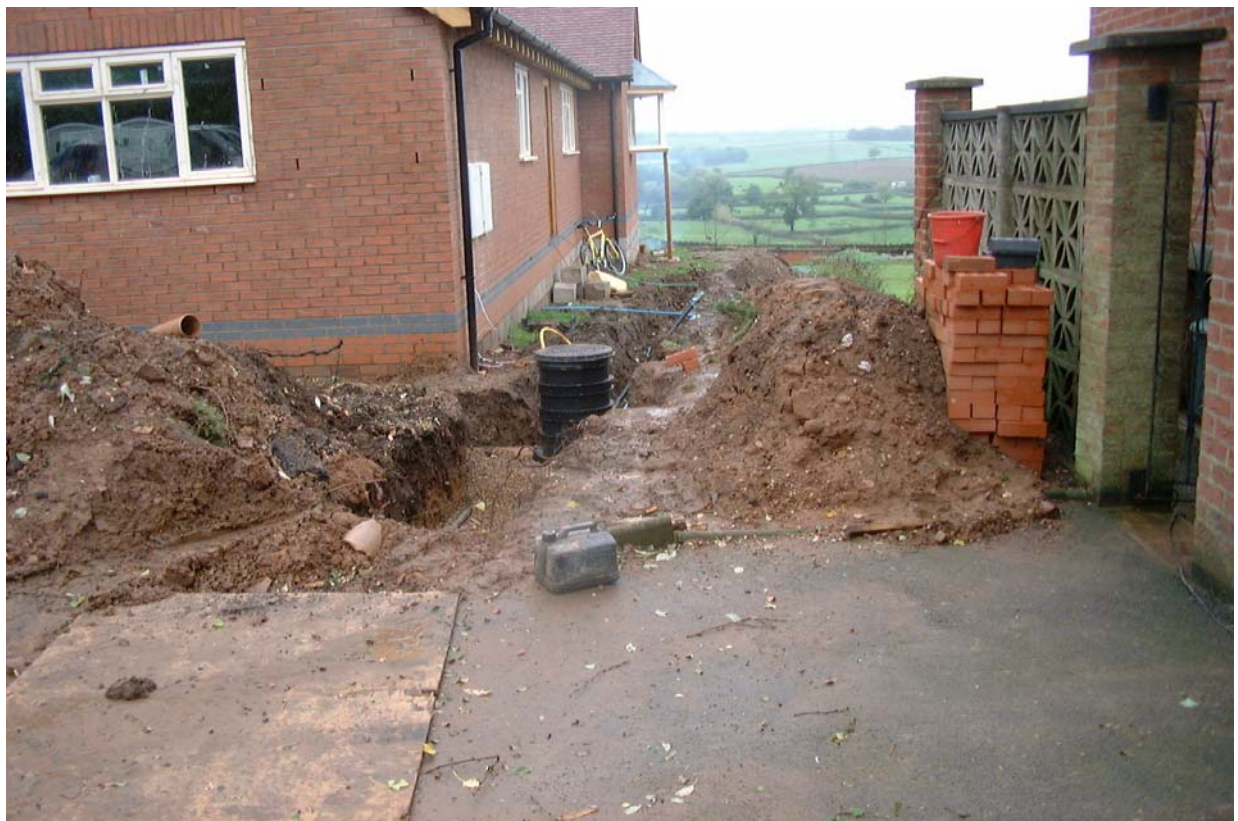
Plate 4: The drainage trench running between Glenaber and the new dwelling
