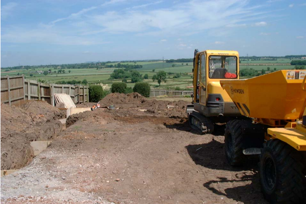
Plate 1: Development area during groundworks, viewed from Church Street
