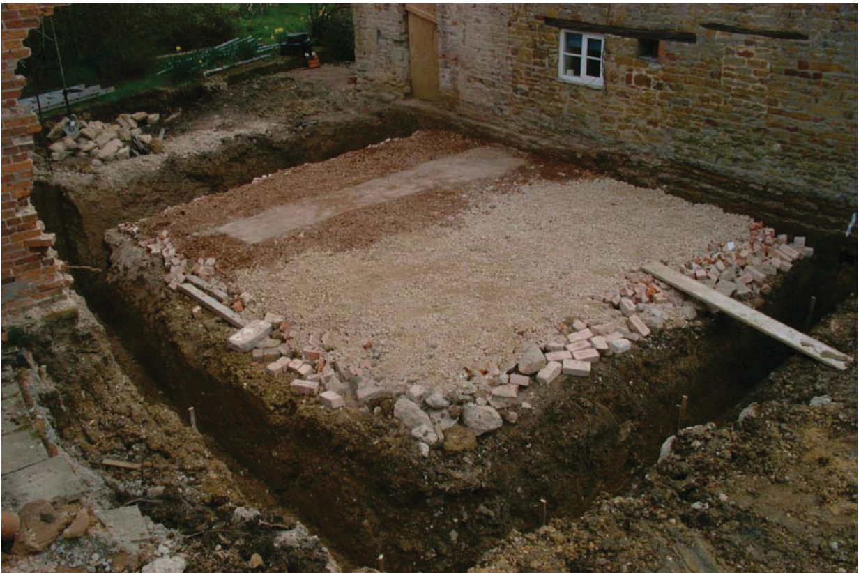
Plate 2: The groundworks for the new extension
