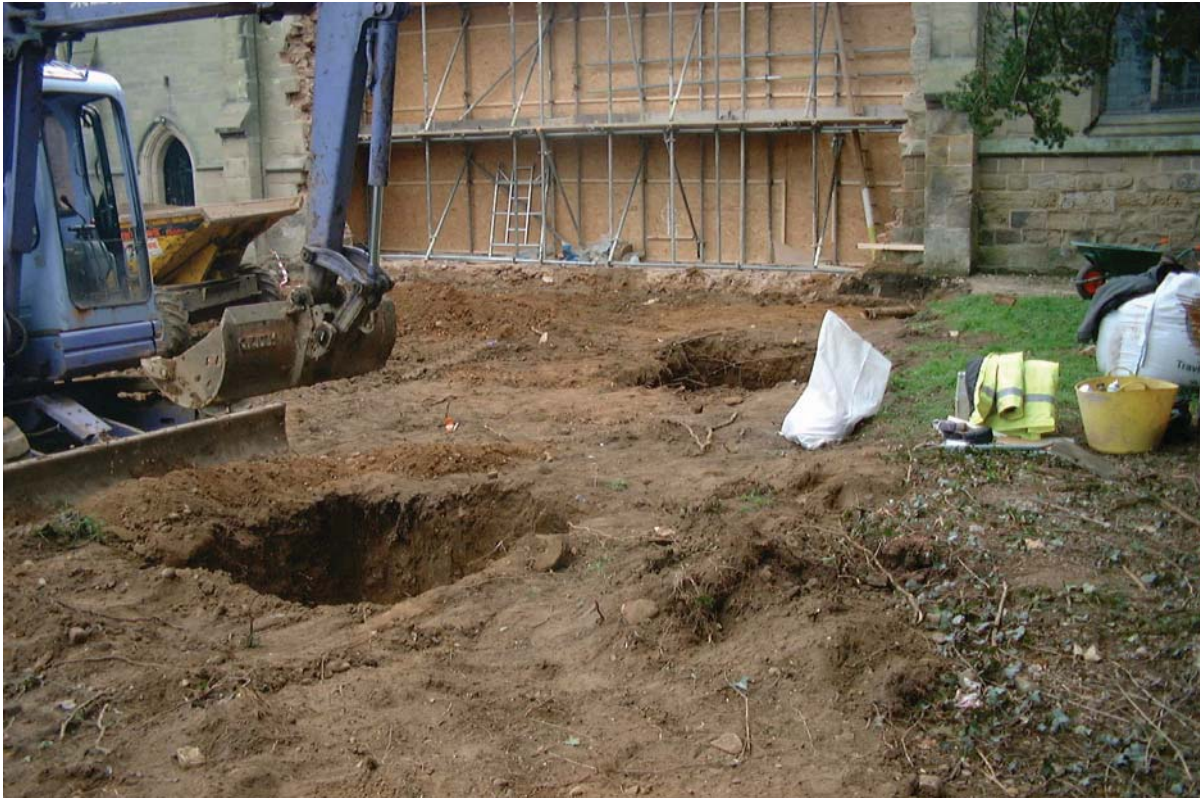
Plate 5: The excavation of the foundation pits
