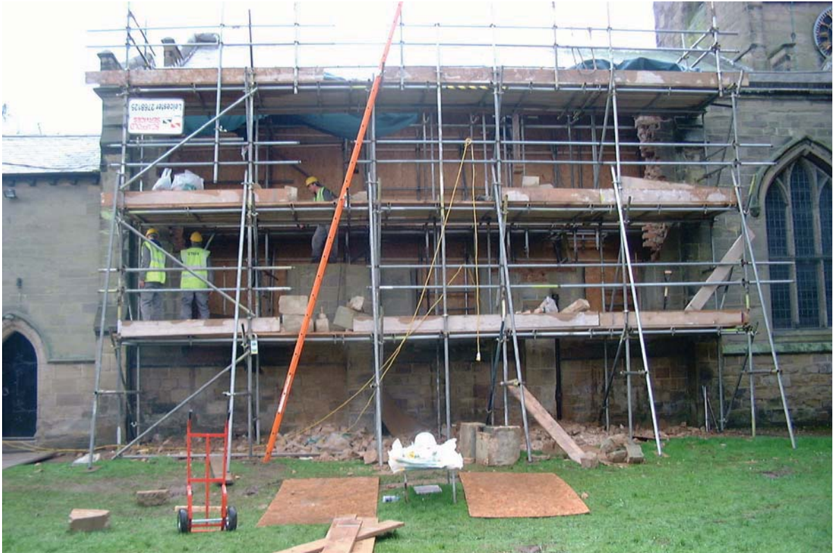
Plate 2: The north wall during dismantling
