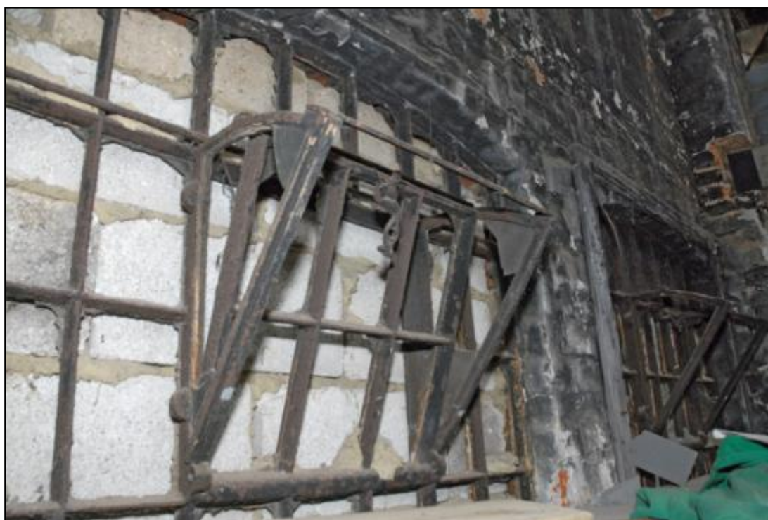
Building 1, ground floor, detail of the window hoppers Fig 29
