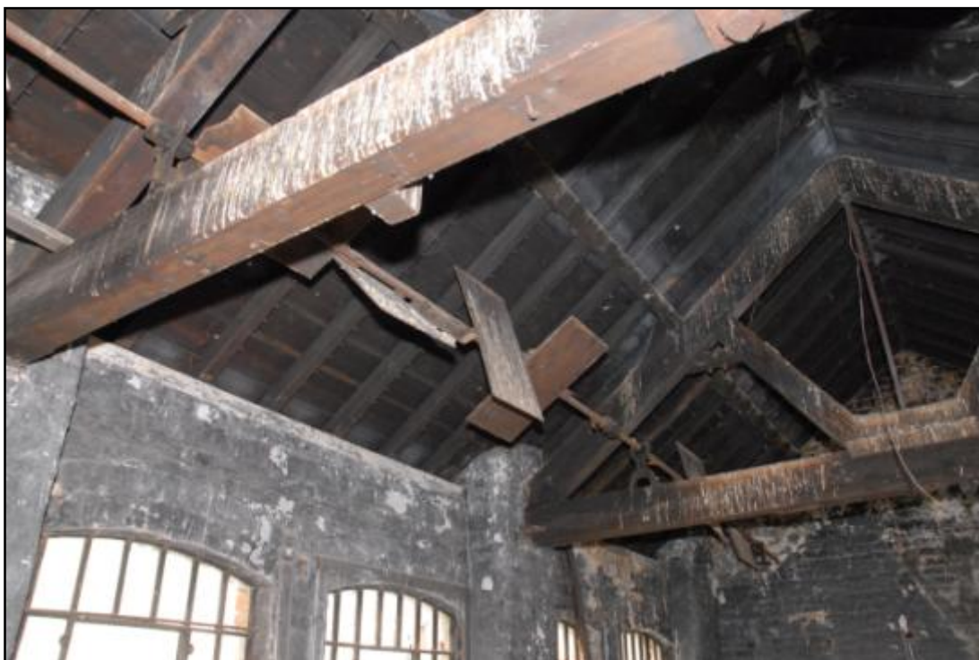
Detail of the drive shaft and “paddles”, looking west Fig 36
