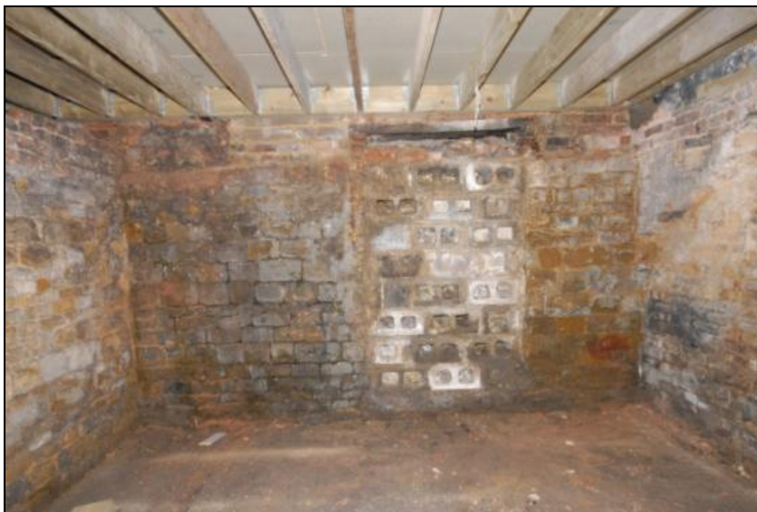
Room B4, showing blocked door, looking south Fig 60
