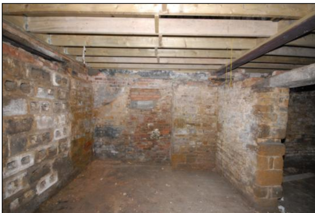
Room B4, showing blocked door, looking west Fig 61
