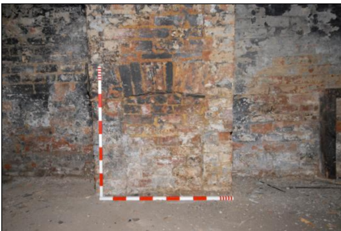
Building 1, detail of the east fireplace Fig 27
