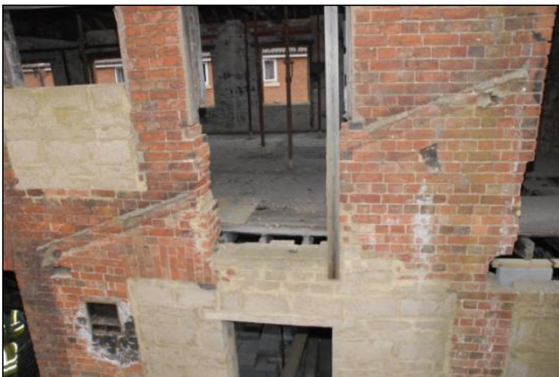
Building 2, scar of former link structure (note square opening at bottom left) Fig 19
