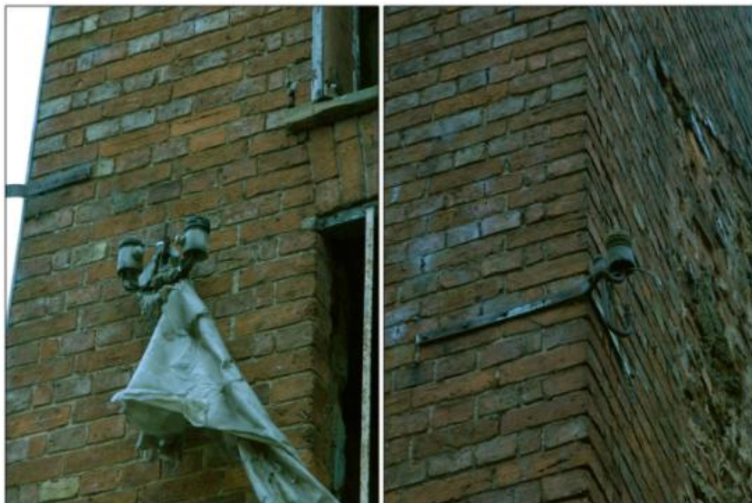
Building 2, north elevation, electrical fittings Fig 22
