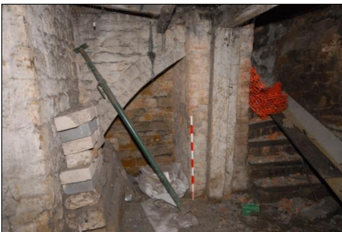
Relieving arch adjacent to basement stair Fig 51
