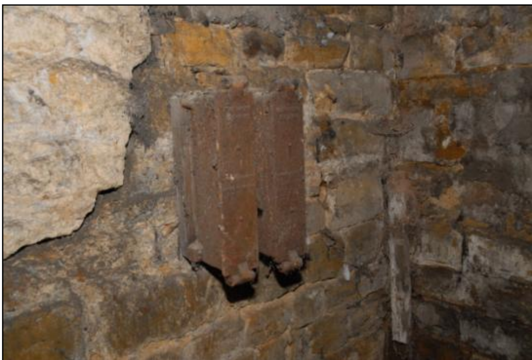
Room B2, detail of the electric box Fig 57
