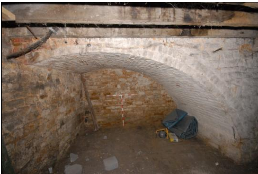
Relieving arch beneath the main stair Fig 52
