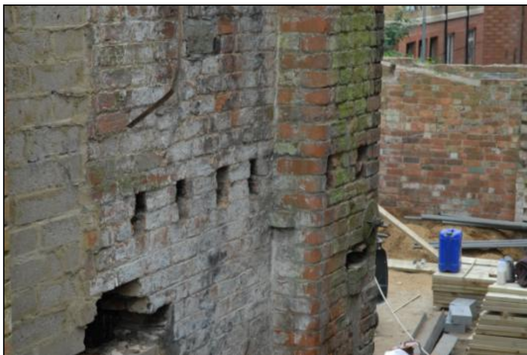
Building 1, north elevation, beam slots Fig 21
