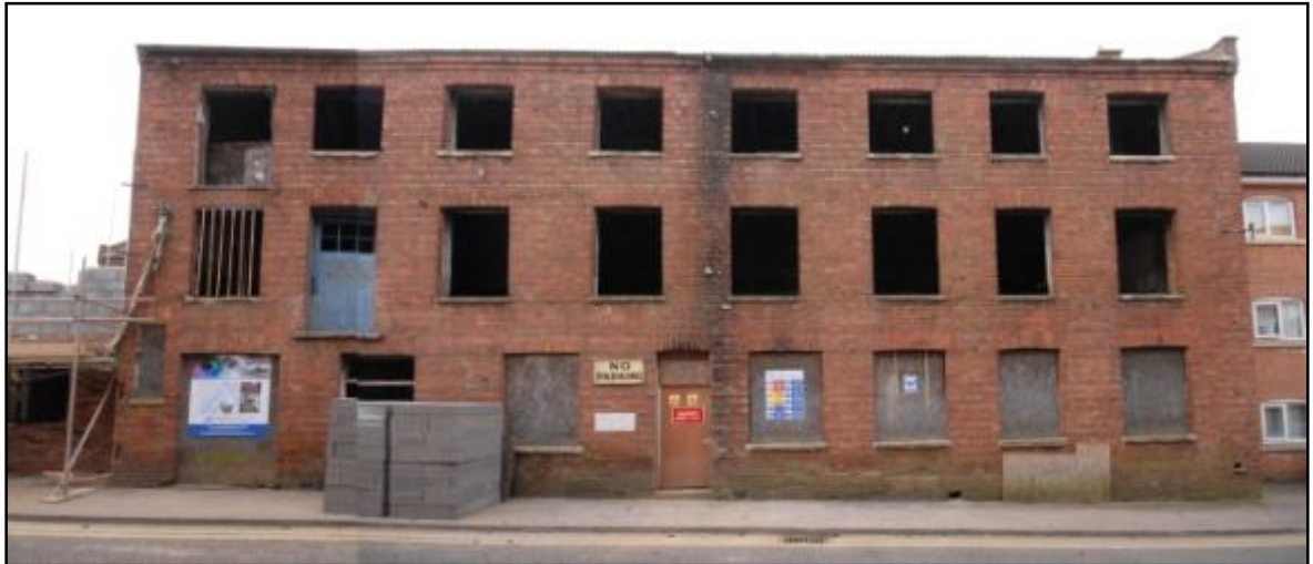
North elevation, Building 2 (Photocomposite), looking south Fig 10
