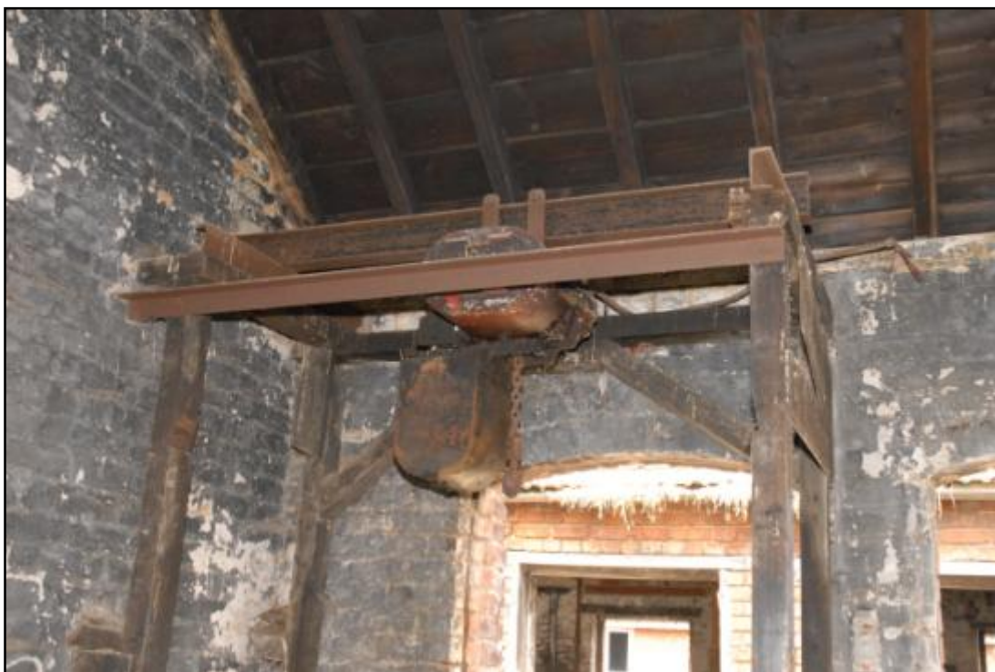
The top of the lift shaft Fig 40
