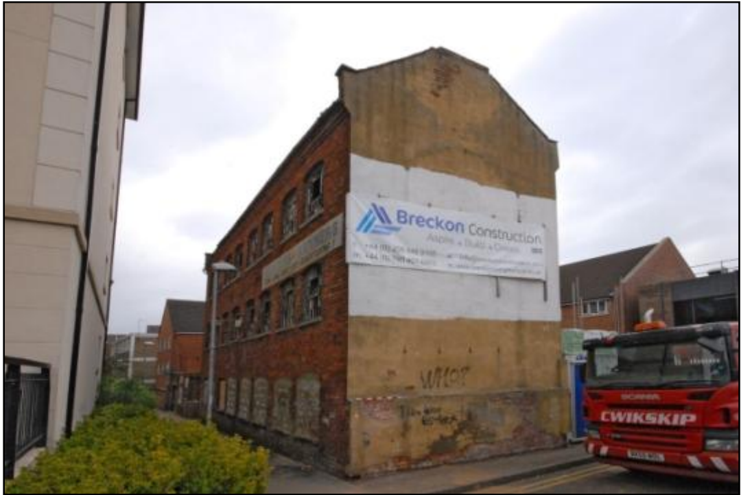
South and east elevations, Building 1, looking north-west Fig 12
