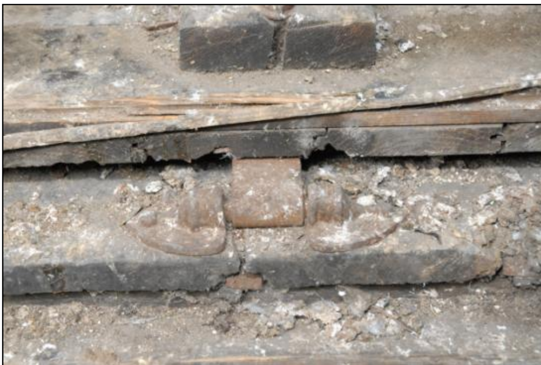
Detail of the trapdoor hinge Fig 42
