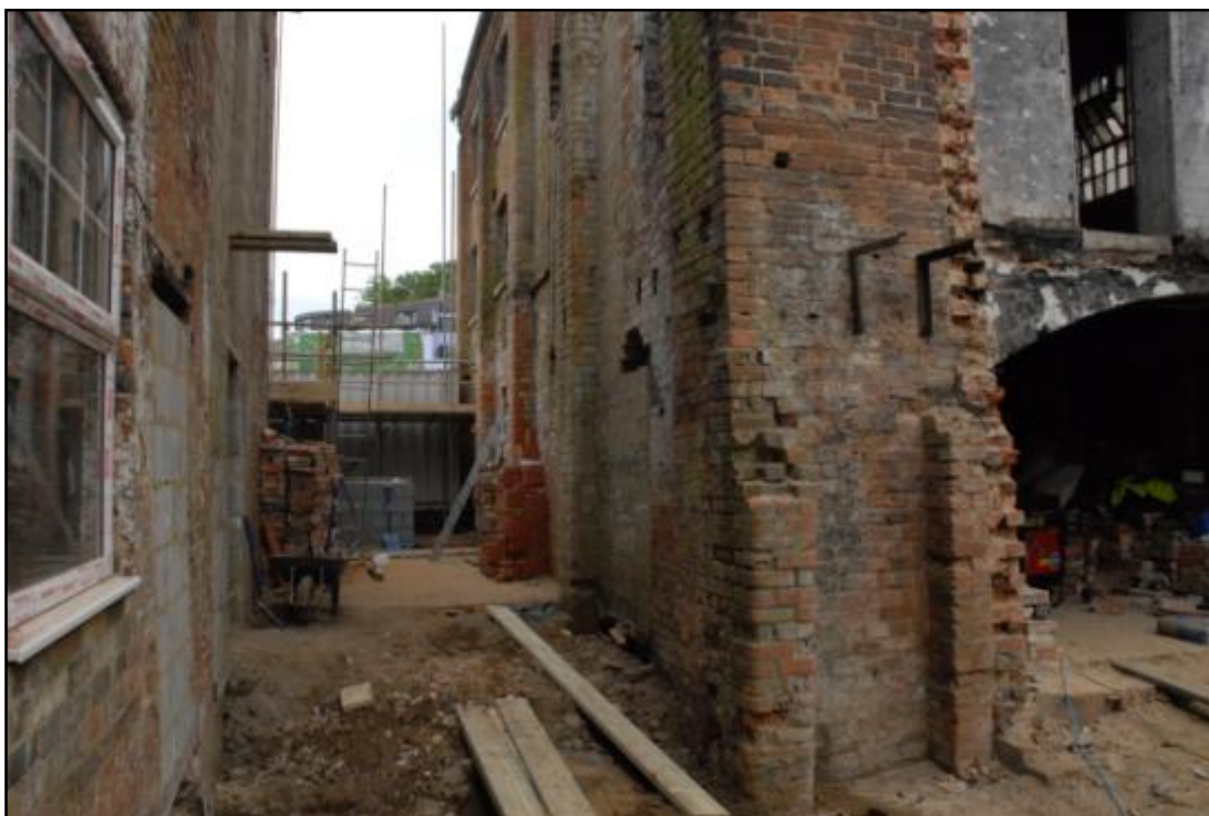
View down the space between the two buildings, looking east Fig 18
