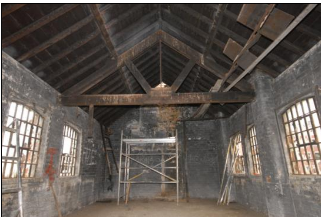
Building 1, second floor, looking east, showing chimney flue Fig 35
