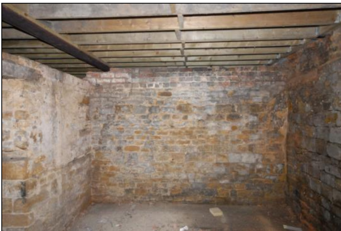
Room B3, the west wall, looking west Fig 59
