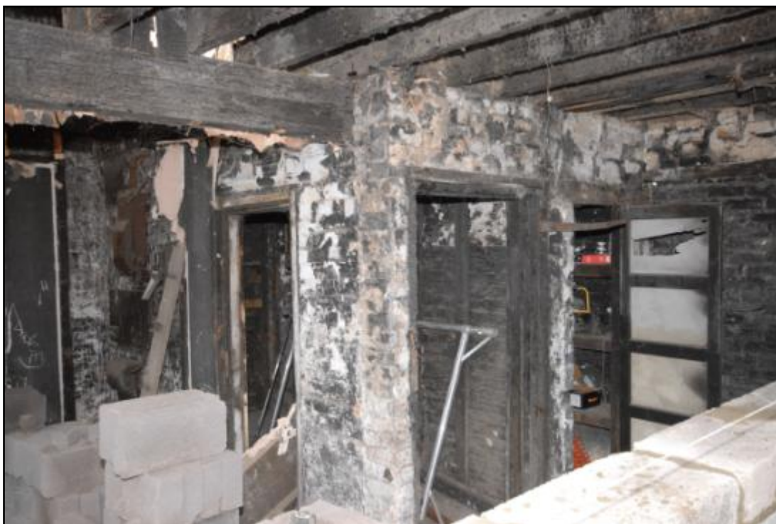
Building 2, ground floor, the lobby and stair Fig 44
