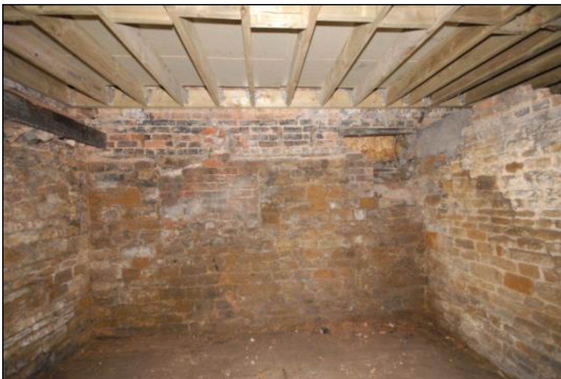
Room B3, blocked light wells, looking north Fig 58
