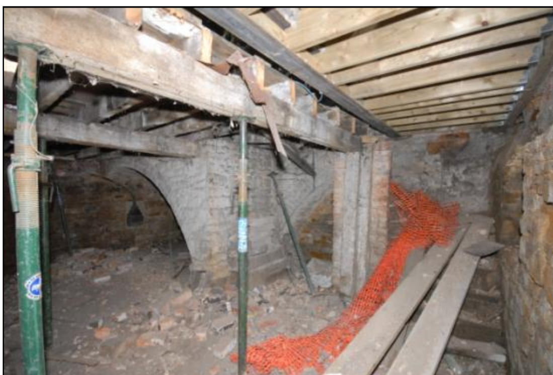
Building 2, Room B1, looking east, showing the stair down and relieving arches for the stair above Fig 49
