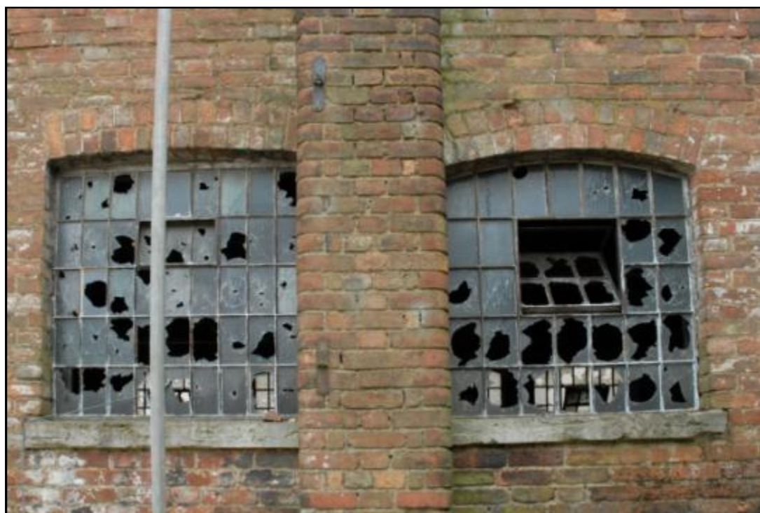
Building 1, north elevation, different window types Fig 23
