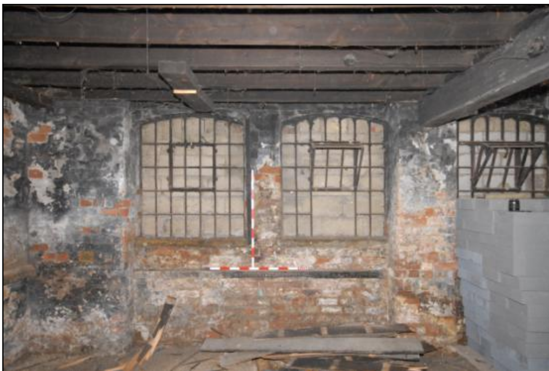
Building 1, ground floor, south wall Fig 28
