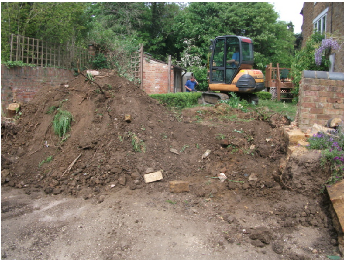
The groundworks in progress, looking west from Main Road Fig 4
