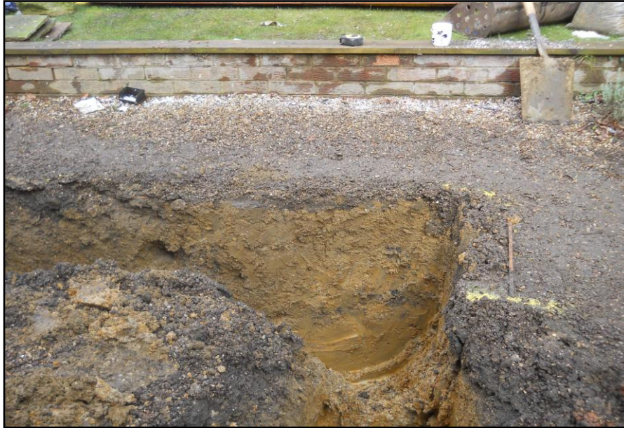
Trench section, looking north-west Fig 4
