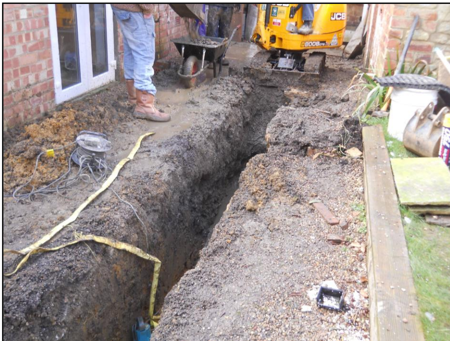
Trench showing back-fill, looking south-west Fig 5
