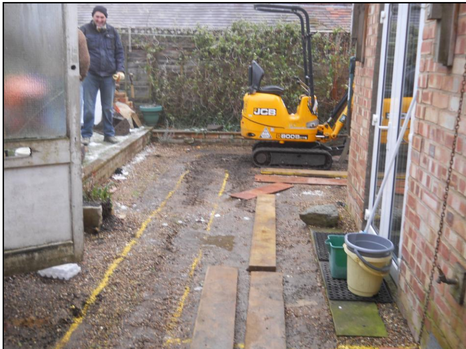
Location of trench, looking north-east
