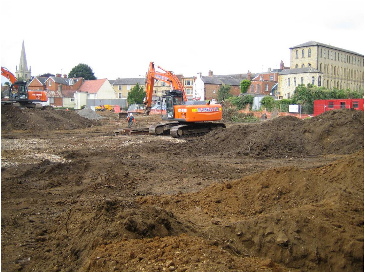
Development site during watching brief, looking west Fig 5
