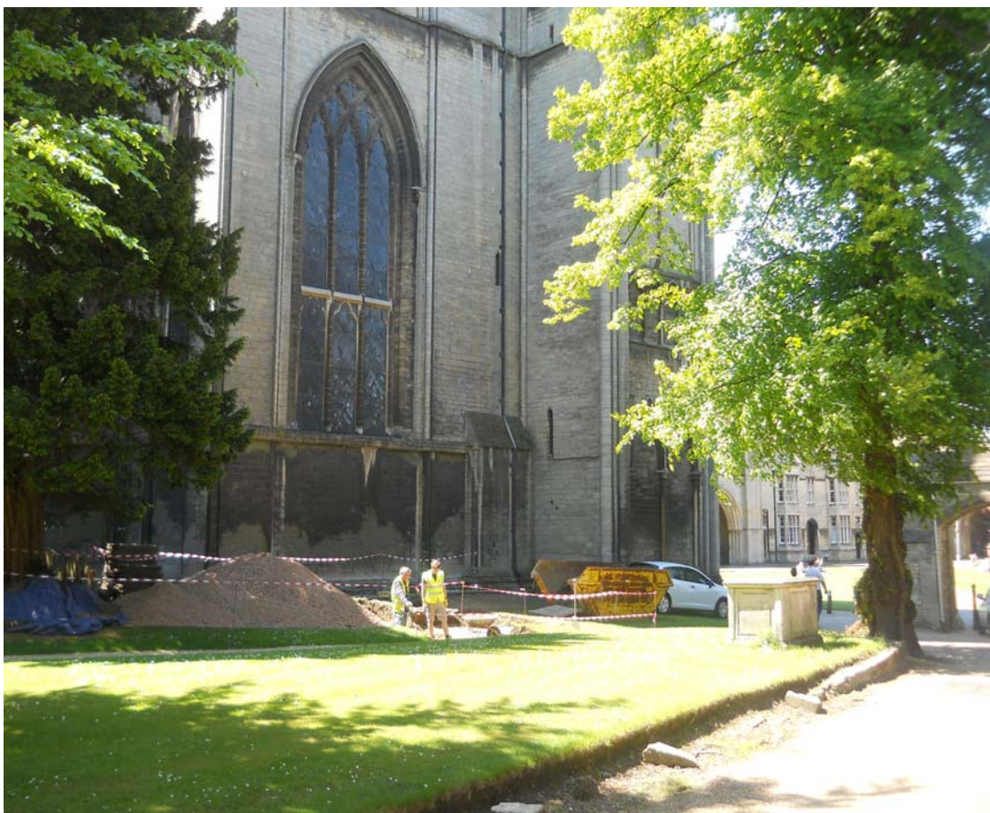
View of watching brief area
