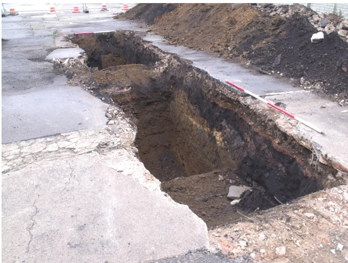
Trench 3, looking south-east Fig 4
