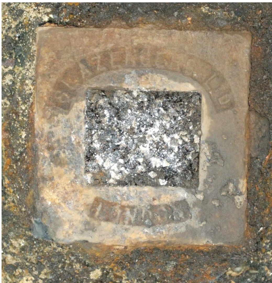
Cast-iron socket formerly containing a post that held up a tennis net (dimensions 120mm x 120mm) Fig 4
