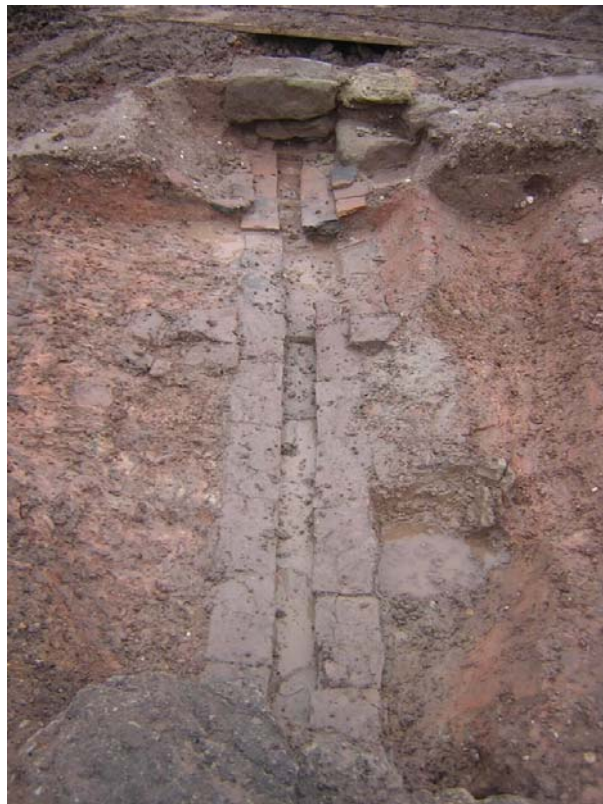
Plate 12: Tile lined drain – looking east
