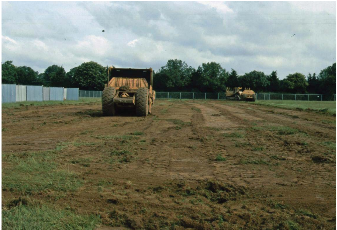
Box scrapers removed the topsoil in the area of future pitches Fig 5
