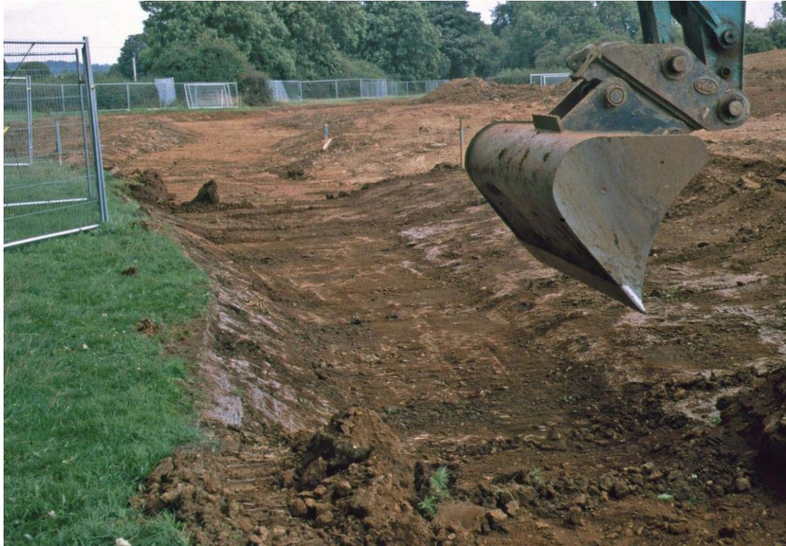
North swale excavated under a controlled watching brief Fig 4
