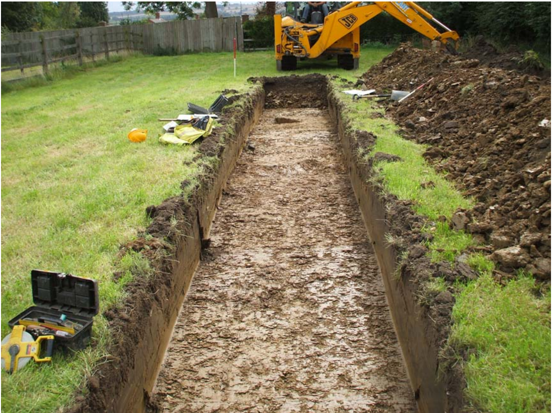
Fig 5 Excavated trench, looking south
