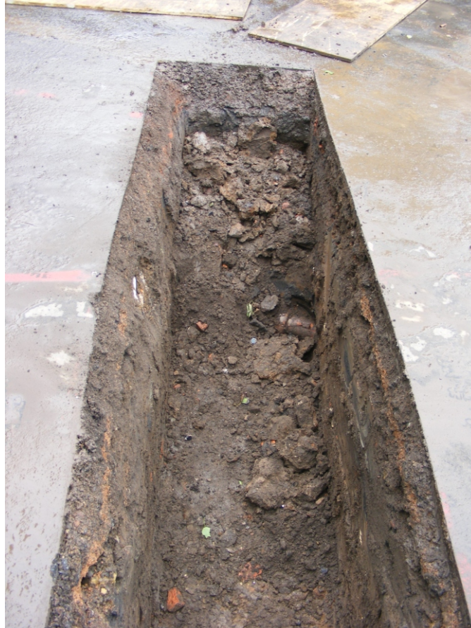
Fig 5: The northern end of the initial trench, showing services at base
