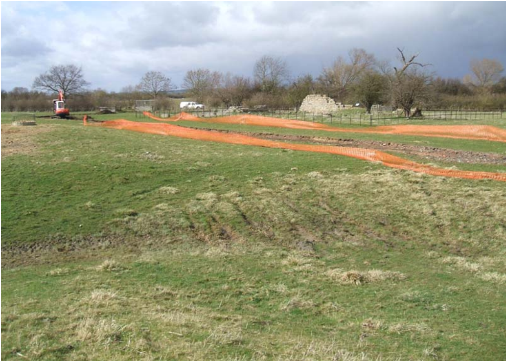
Fig 15: General view of footpath under construction
