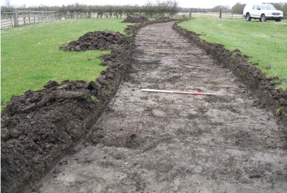
Fig 18: General view of the footpath northern spur
