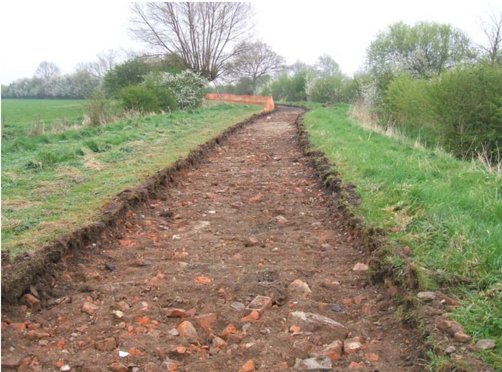
Fig 16: Farm track rubble exposed
