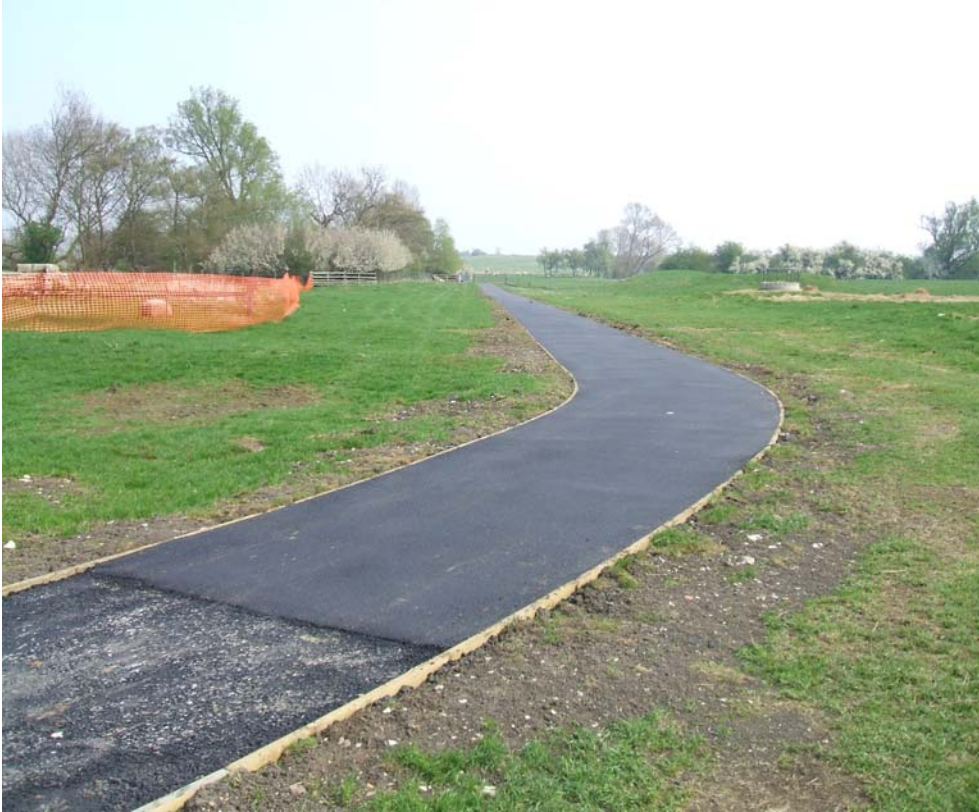
Fig 17: Partially completed footpath
