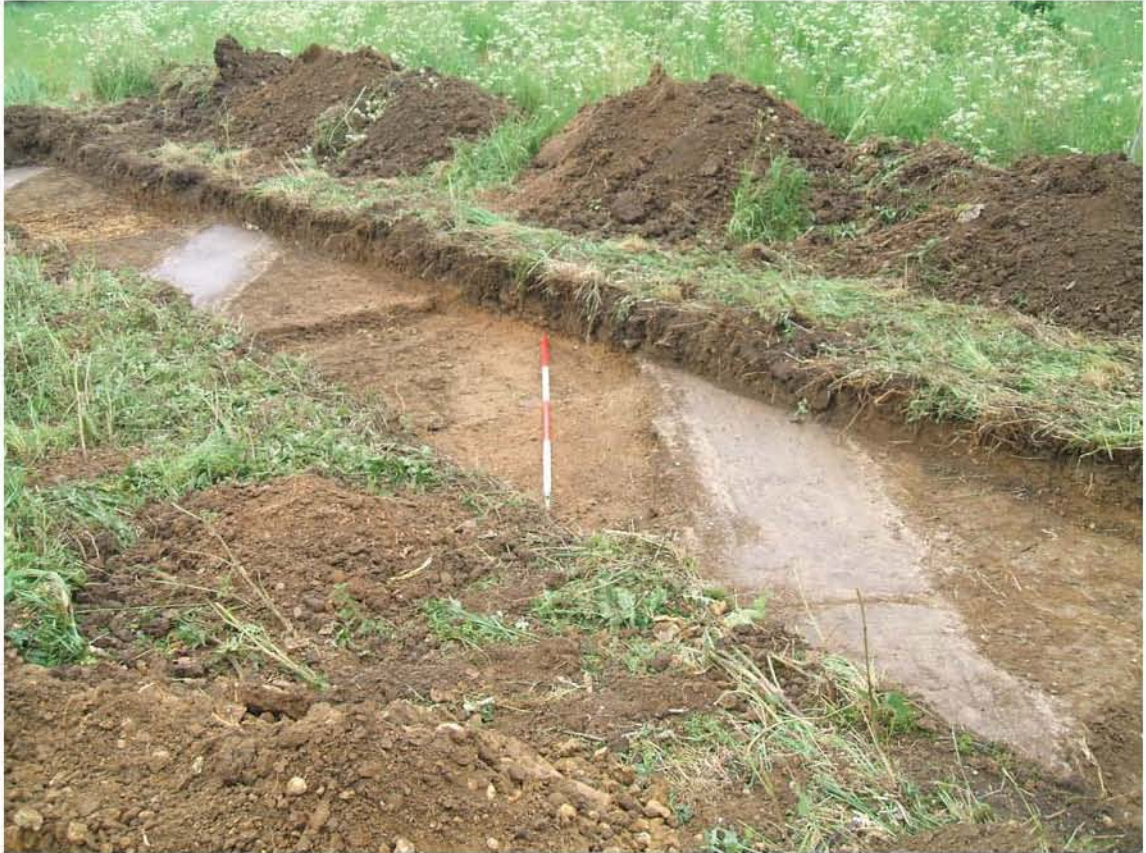
Concrete foundations in the southern end of Trench 1, looking east
