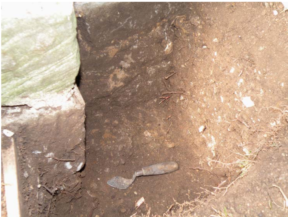
Cut for buttress foundation Fig 4
