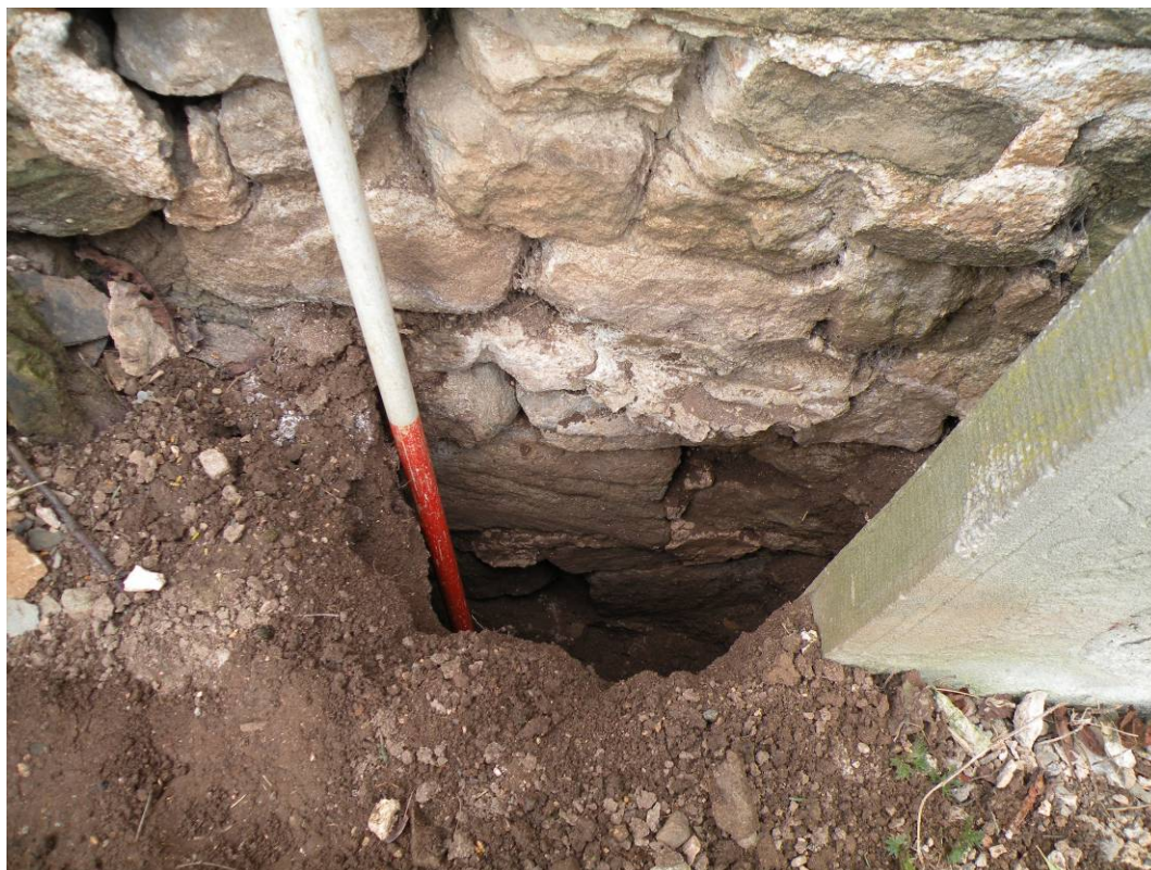
Test pit 2 showing character of the east wall of the church
