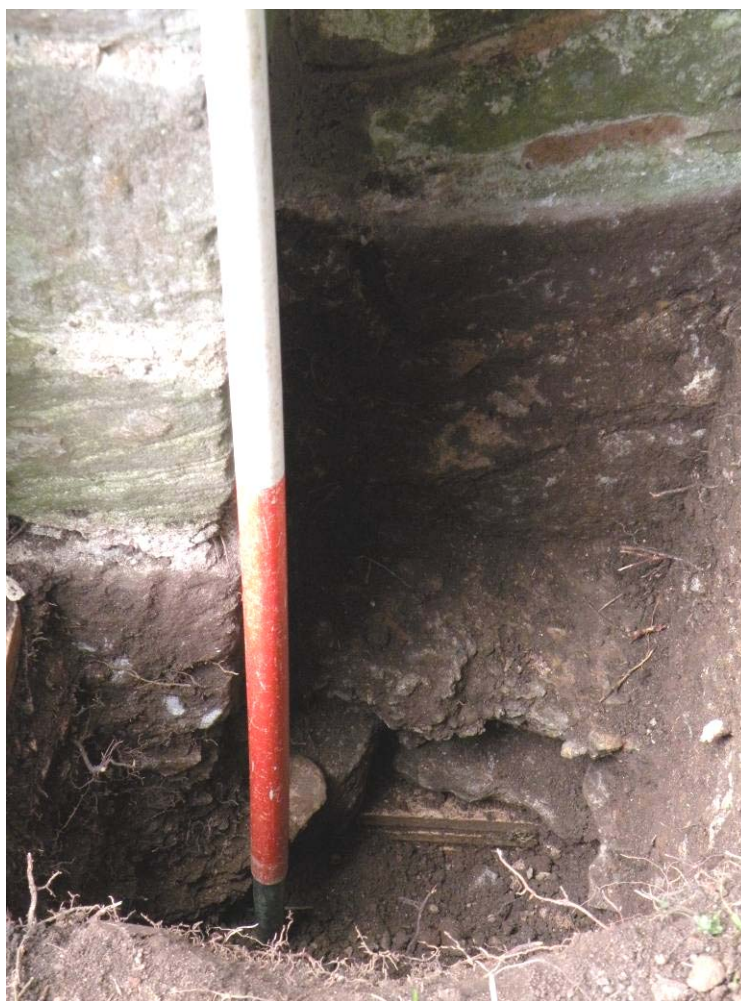
Base of buttress foundation showing glazed brick/tile Fig 5
