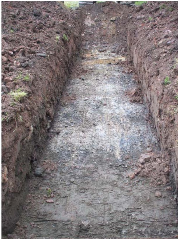
View of Trench 6, showing yard surface, looking south
