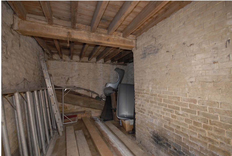
The Store with the brick dividing wall
