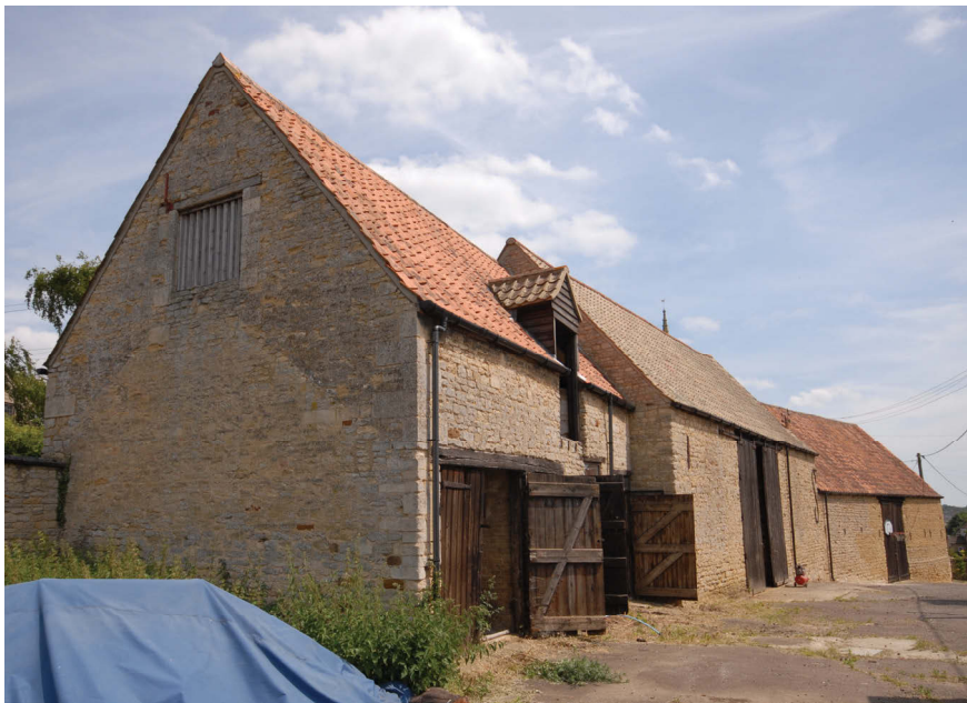
The range of barns, looking south-east
