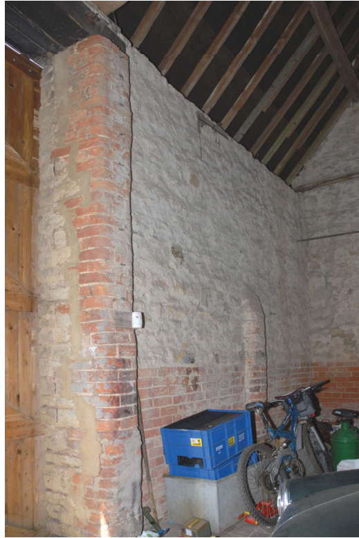
Barn 1, west corner Fig 10
