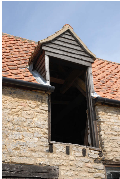
The pitching door and gablet in the hayloft roof
