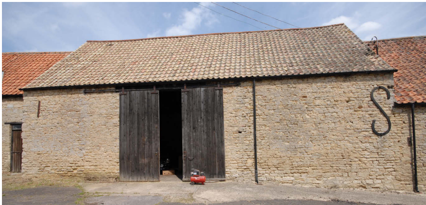
Barn 1, south-west elevation
