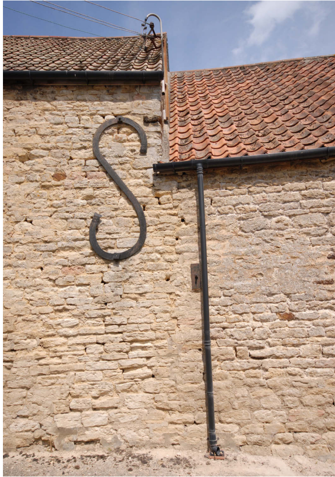
The join between Barns 1 and 3, south-west elevation Fig 22
