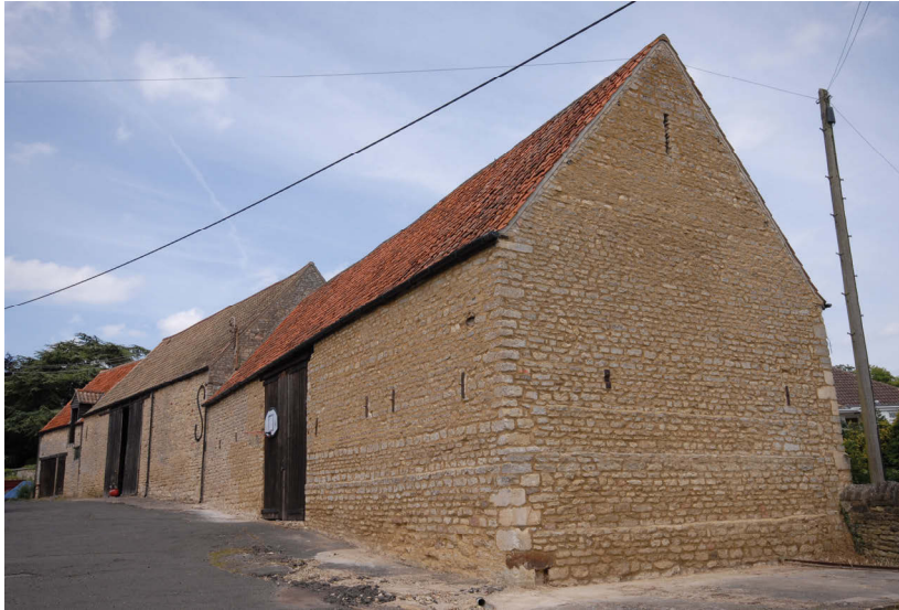
The southern corner of Barn 3 Fig 21
