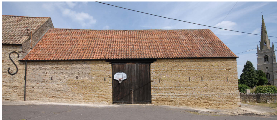
Barn 3, south-west elevation
