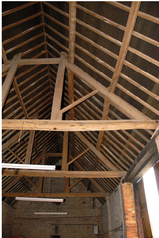
The roof timbers and felting to Barn 1 Fig 11
