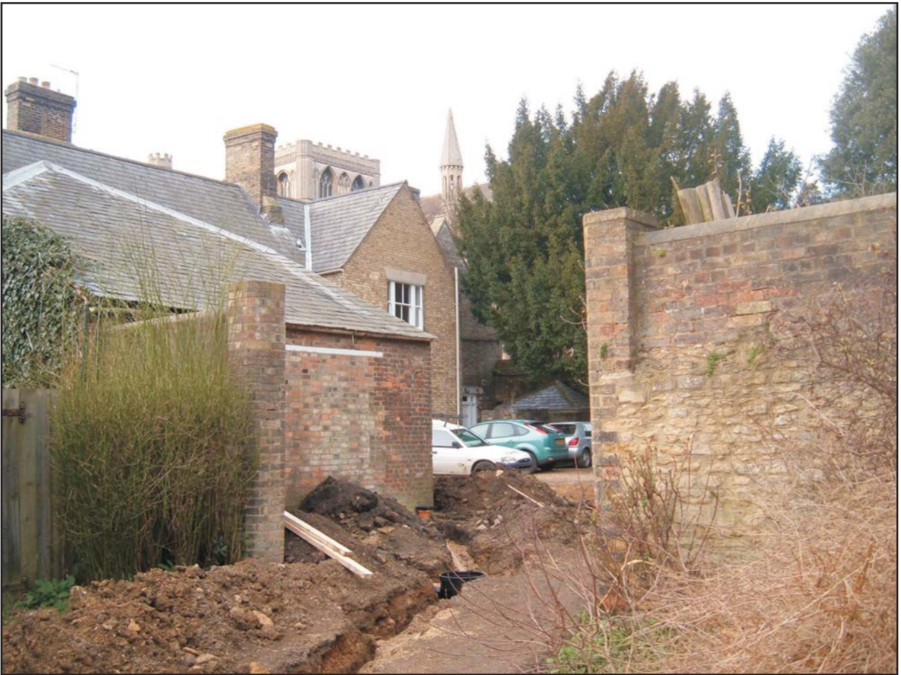
General view of trench 3, looking north-west Fig 5
