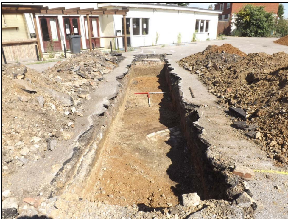
Trench 2, looking east,
