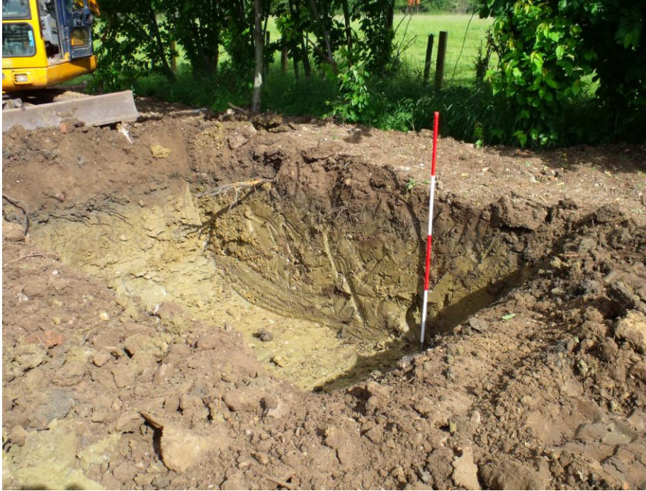
The hole for the sewerage tank after excavation
