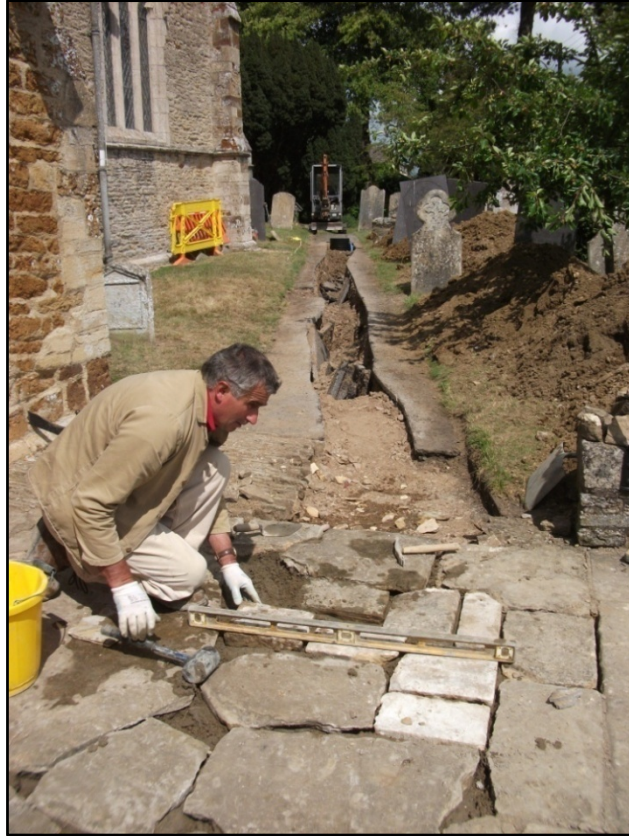
The service trench, looking east Fig 5
