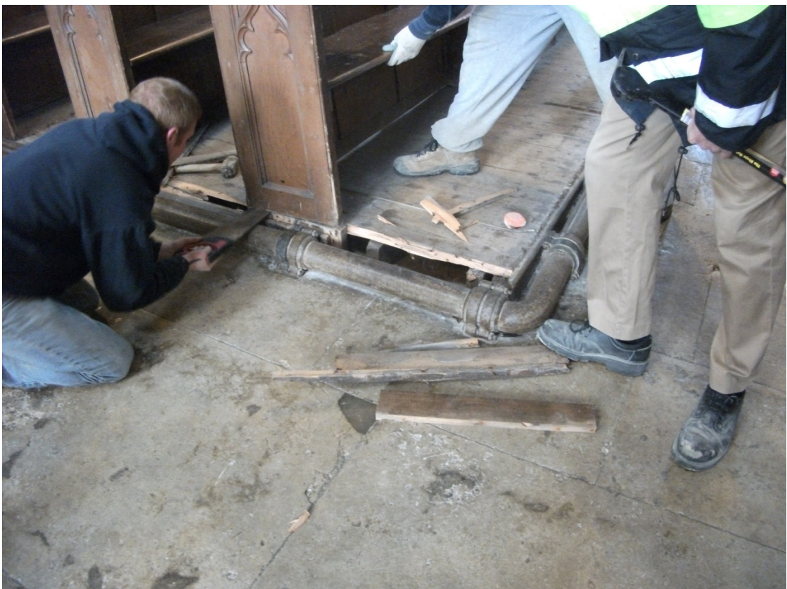
The removal of the pews Fig 5
