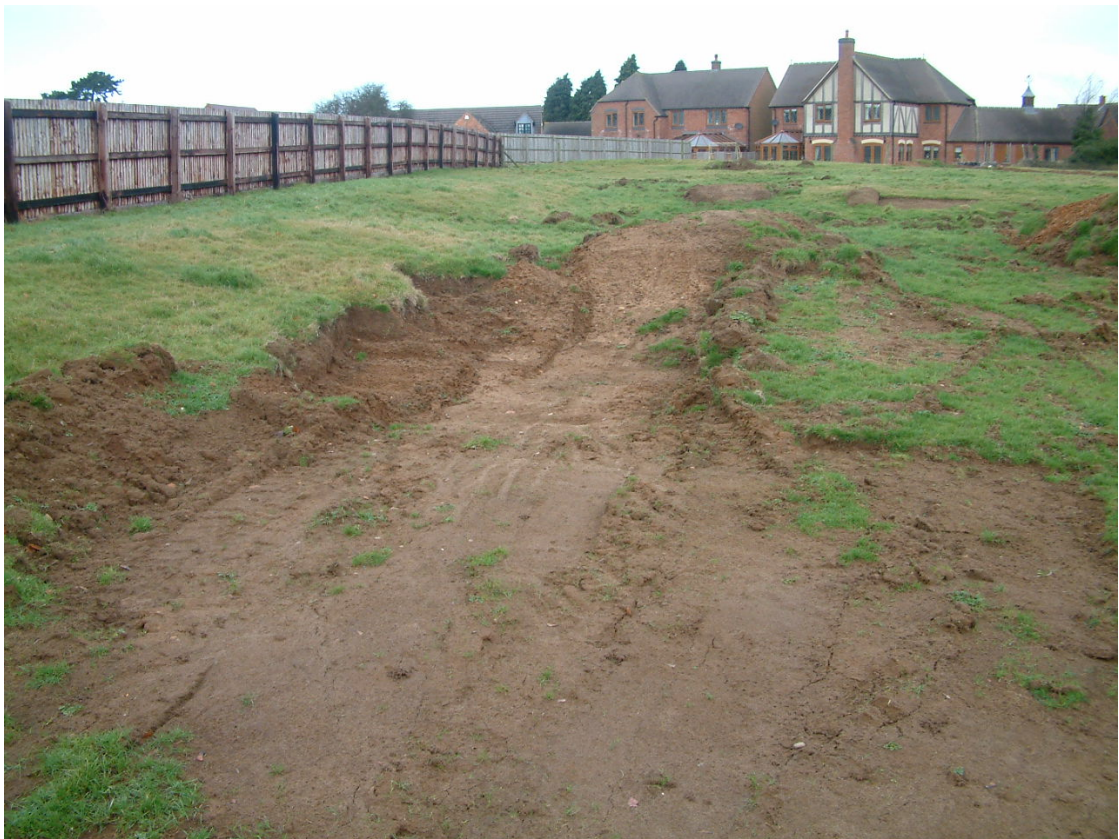
General site view, looking north Fig 5
