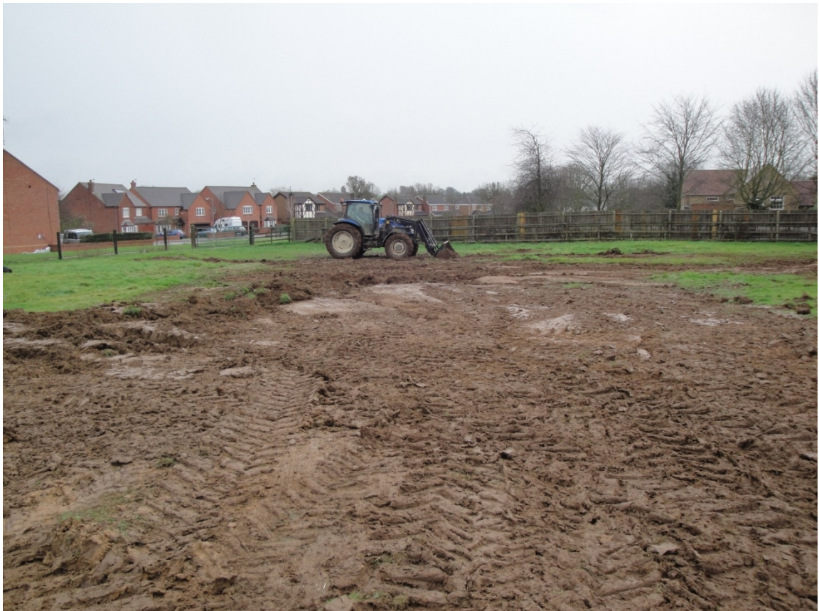
Reinstatement of site, looking south-east Fig 12
