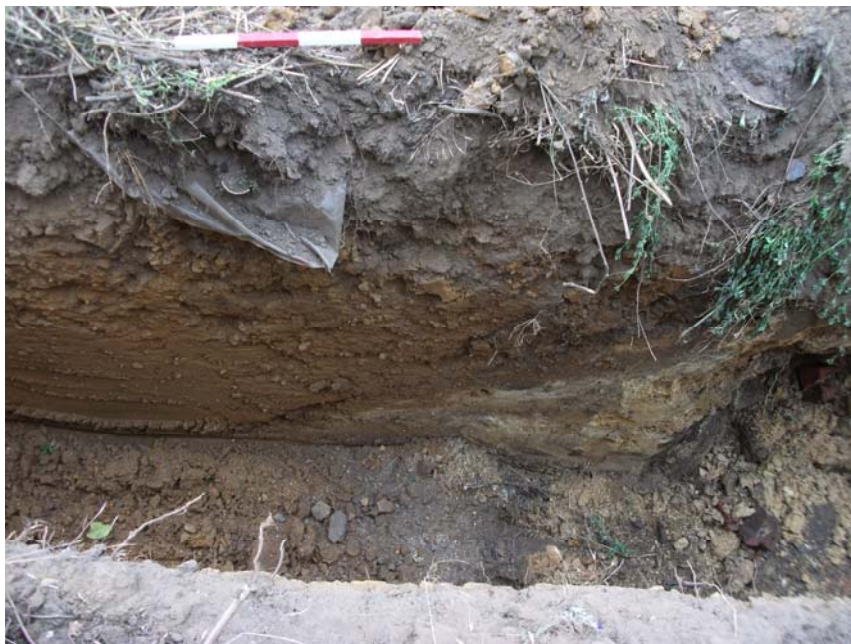
West side foundation trench, section showing natural sand and ironstone, and collapsed brickwork, looking north-west Fig 5
