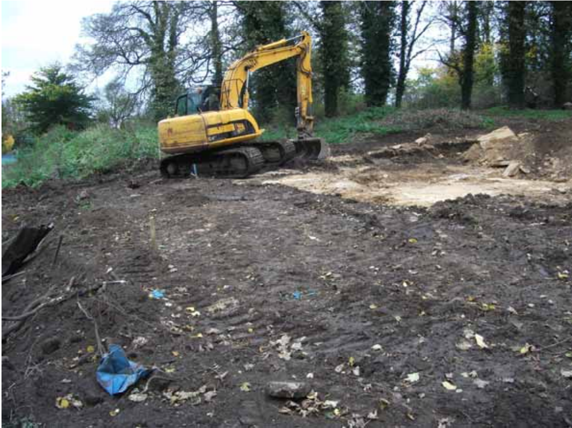
The groundworks in progress, looking north-east Fig 5
