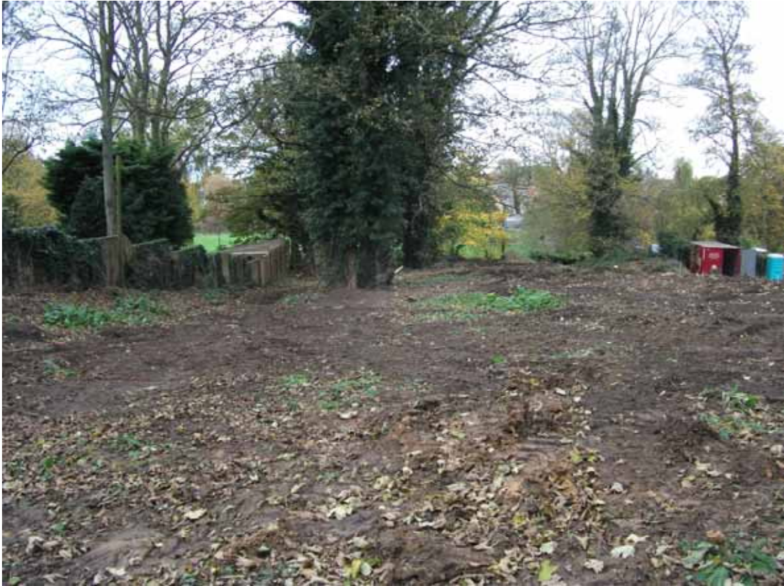
The development area at the start of groundworks, looking north-west Fig 3
