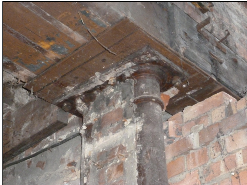
Iron column between the shop fronts of 5 and 7 Sheep Street
