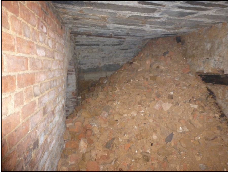
Cellar 3 interior, looking east
