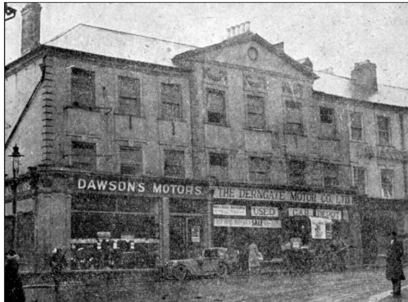
Building making up 1, 3 and 5 Sheep Street (no 5 is at the far right of the photograph) Fig 3
