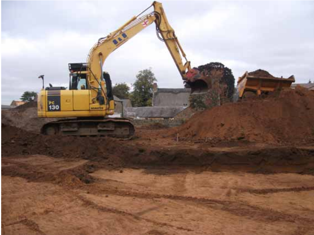
The groundworks in progress, looking east Fig 4
