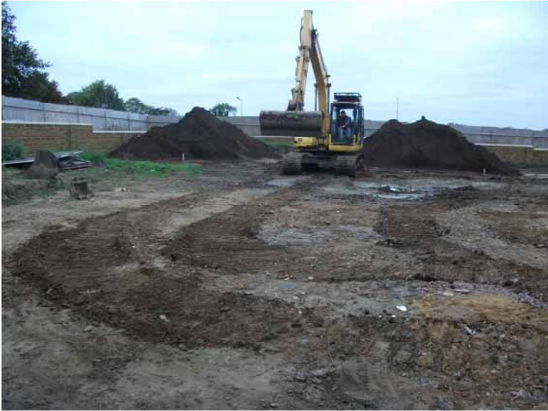
The development area at the start of groundworks, looking west Fig 3
