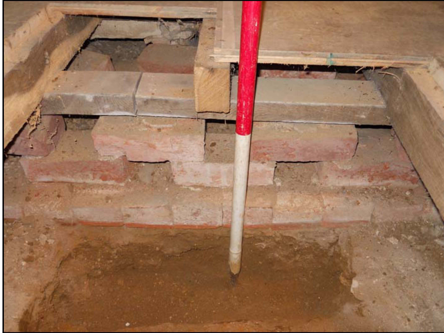
Section showing the floor construction in Test Pit 2, looking south-west Fig 8
