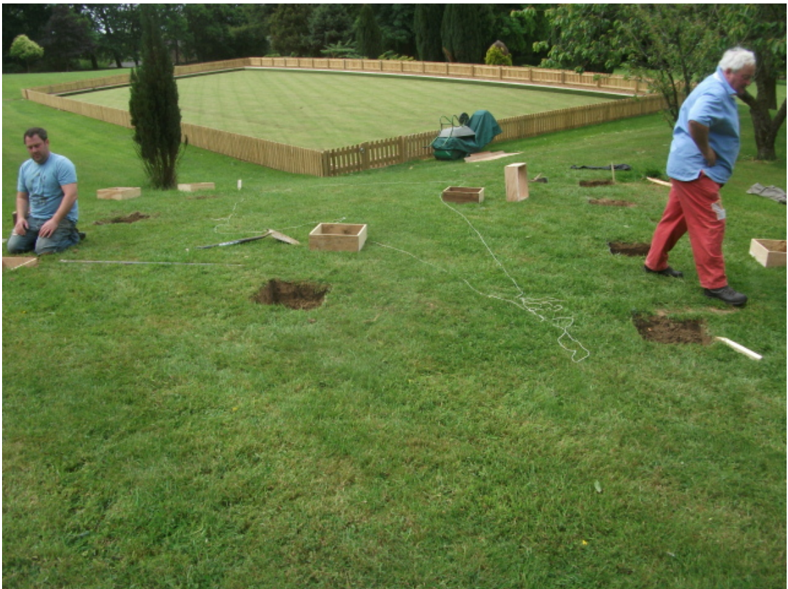
General view of the groundworks, looking south Fig 4
