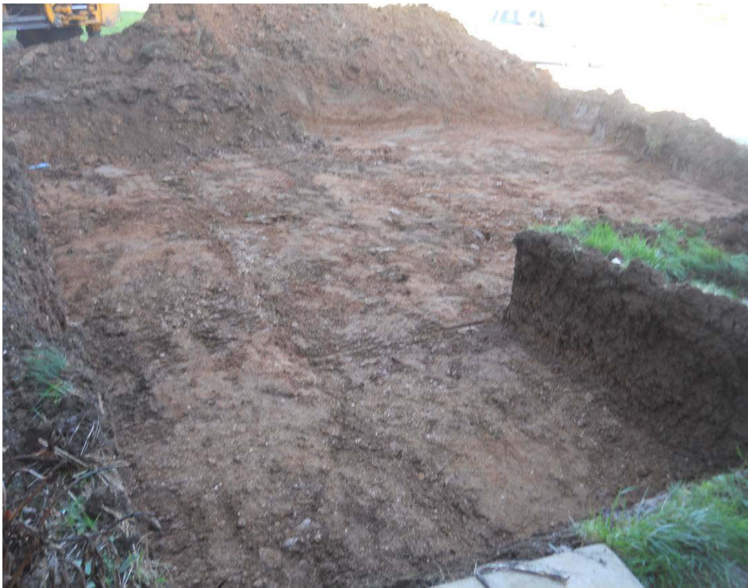
Excavated area, looking north
